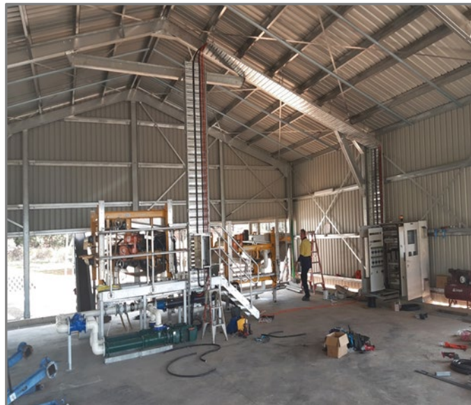
Figure 7: Installation of Belt Filter Press
