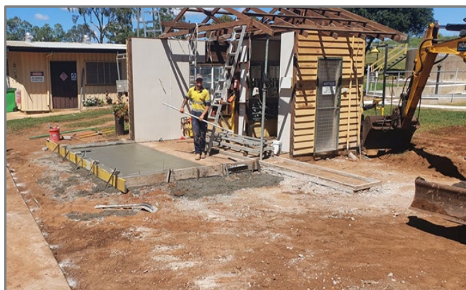
Figure 11: Laying of new extension slab and removal of old building
