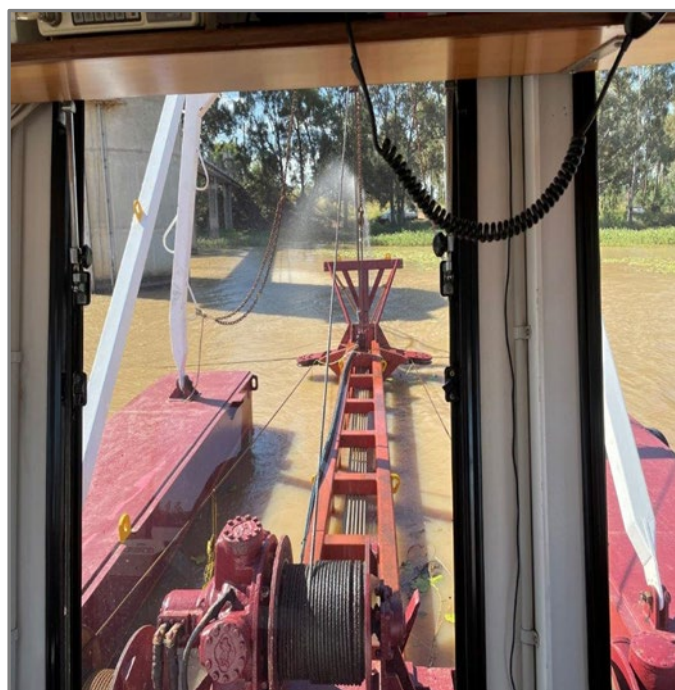
Figure 2: The barge in operation dredging the dam
