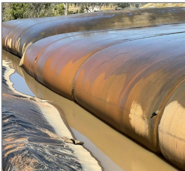
Figure 3: Geo bags being filled
