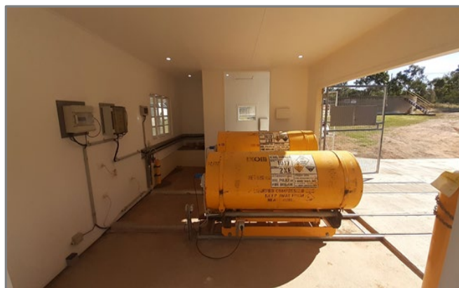
Figure 13: Chlorine cylinders installed in the new building
