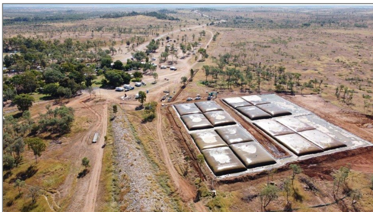
Figure 5: Geo bags have been filled; this will be where they are stored for the next 9 - 12 months
