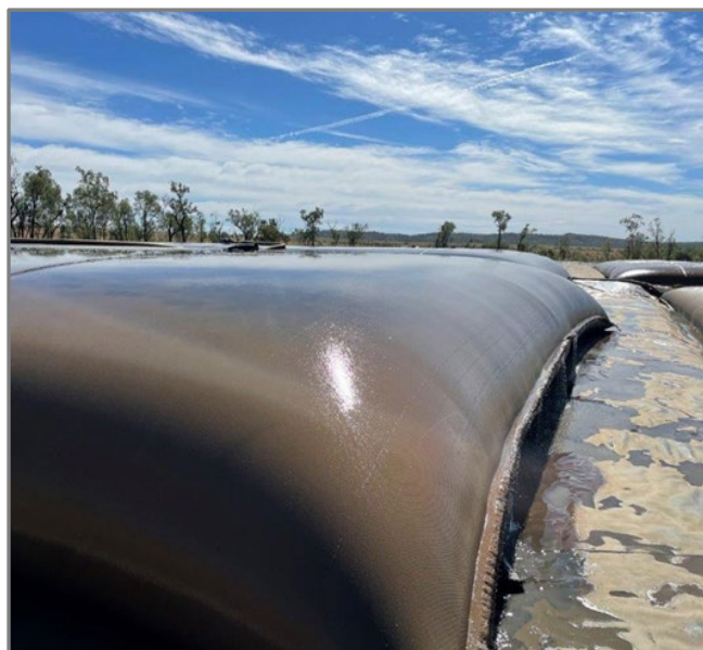
Figure 4: Geo bags being filled
