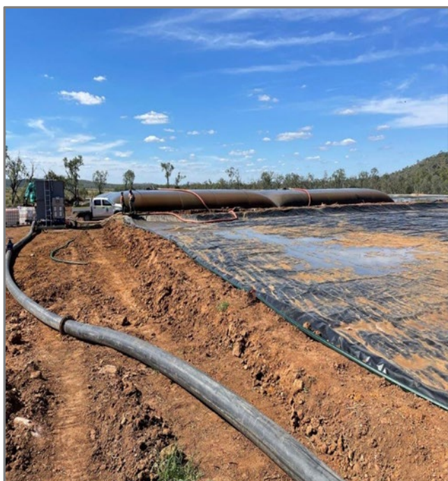
Figure 1: Geo tubes with the extraction pipe in place showing the filling of bags
