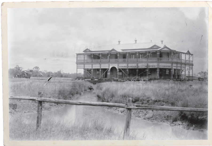
Figure 6: Relocating the Commercial Hotel. Gordon C. Pullar. Source: National Library of Australia.
