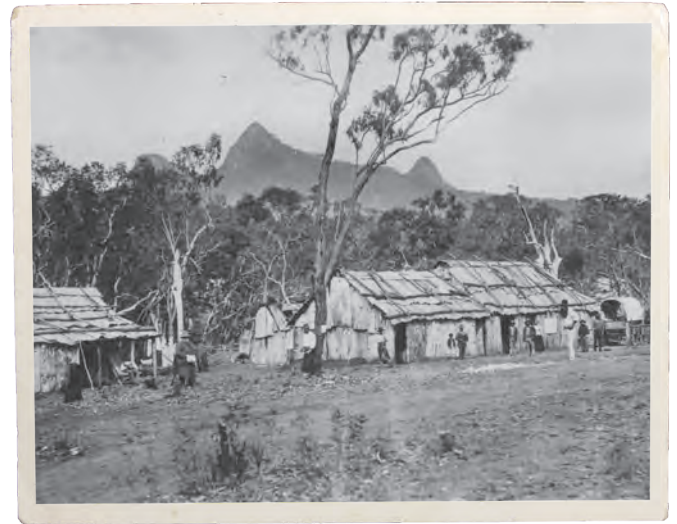
Figure 17: Bark buildings at Mount Britton goldfield, c.1881. Source: State Library of Queensland.
