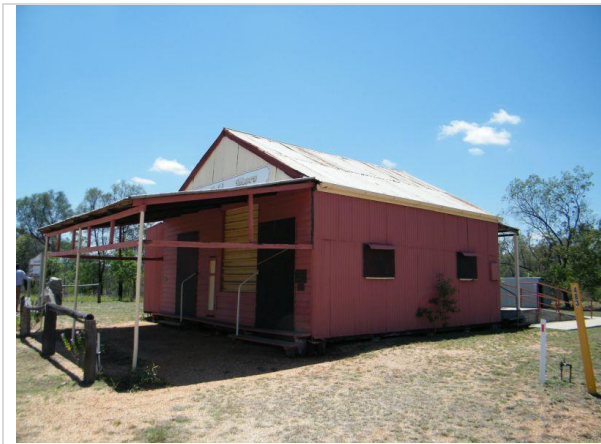
Western and Southern elevations showing cladding and front awning arrangement
