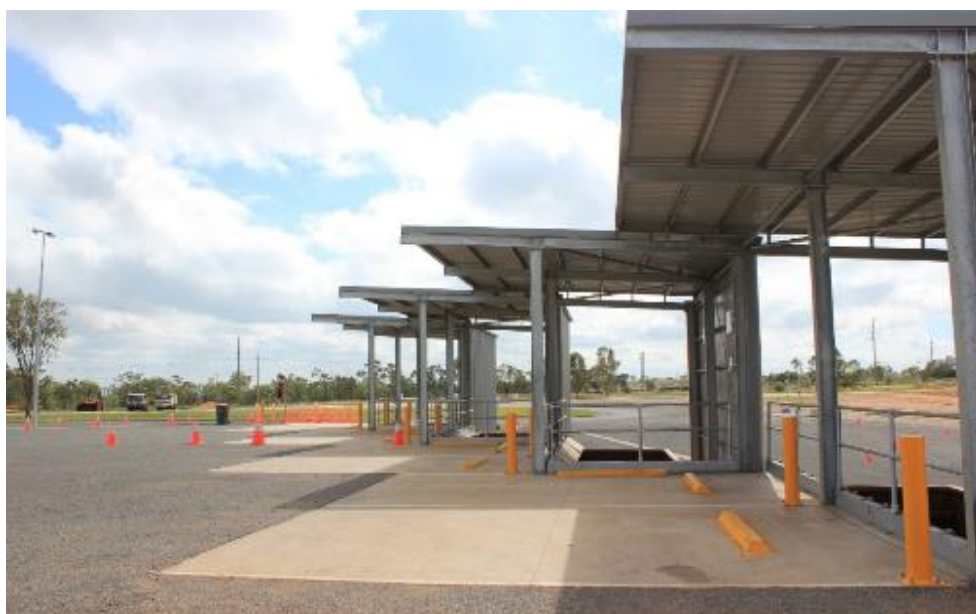
Figure 4-2: Transfer Bays at Moranbah Waste Management Facility
