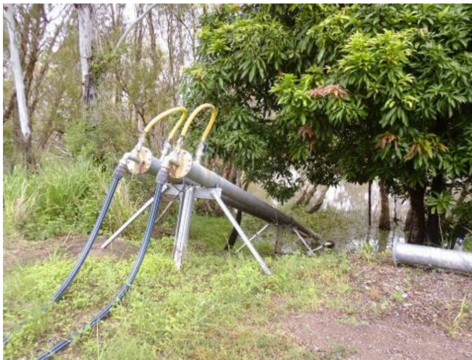
Figure 0-4: Raw Water Pumps at St Lawrence Weir
