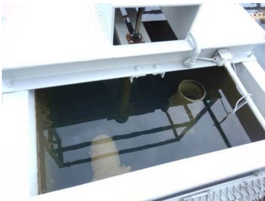
Figure 0-5: Flash Mixer/Flocculation Chamber
