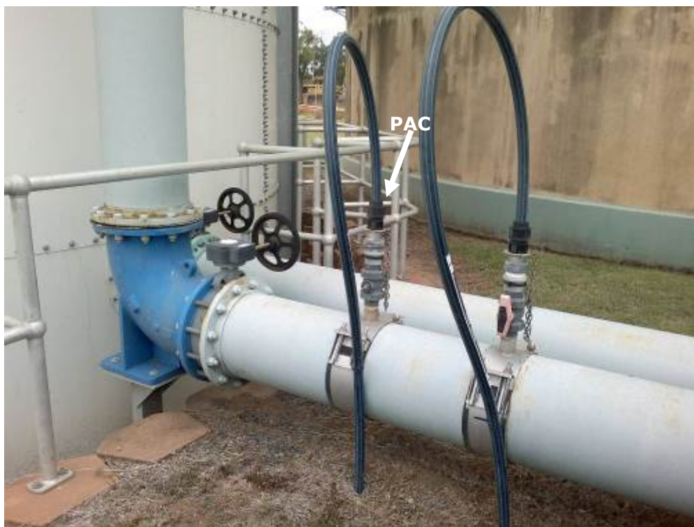
Figure 0-8: Dosing Points on Contact Tank Inlet
