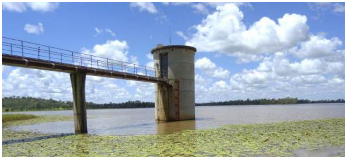
Figure 0-3: Theresa Creek Dam Intake Tower
