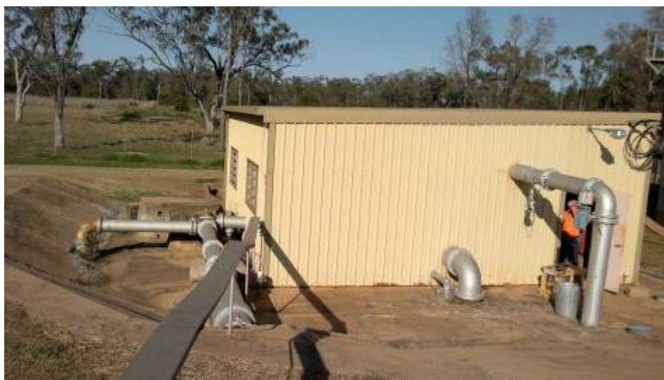
Figure 0-8: High-lift pump rising main (left) and filter backwash line (right)
