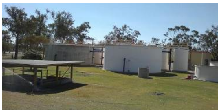
Figure 0-5: Middlemount Clarifiers and Sand Filters
