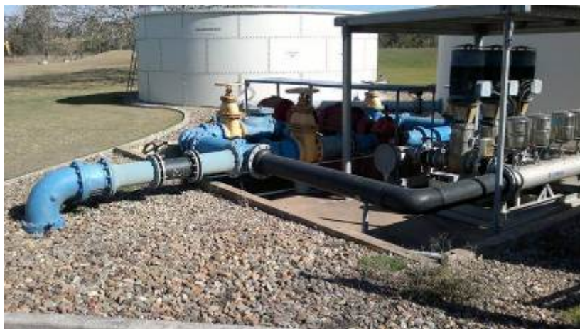
Figure 0-6: Middlemount WTP Lift Pumps
