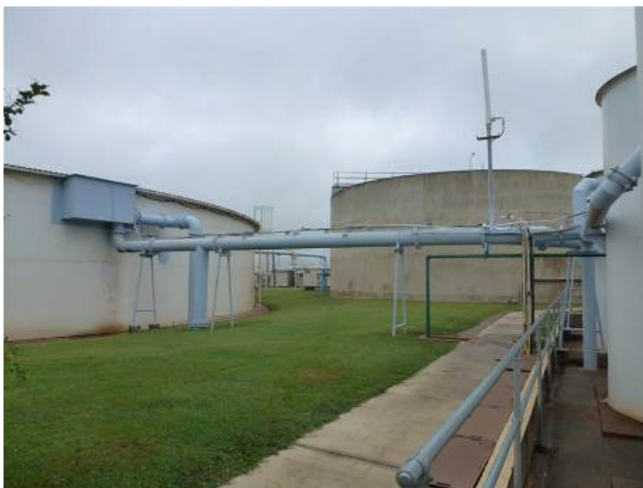
Figure 0-5: Moranbah Filtered Water Line from Bobby WTP into Treated Water Res 1
