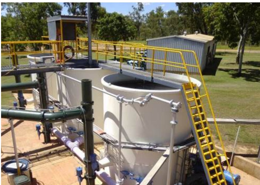
Figure 0-6: Rapid Sand Filters
