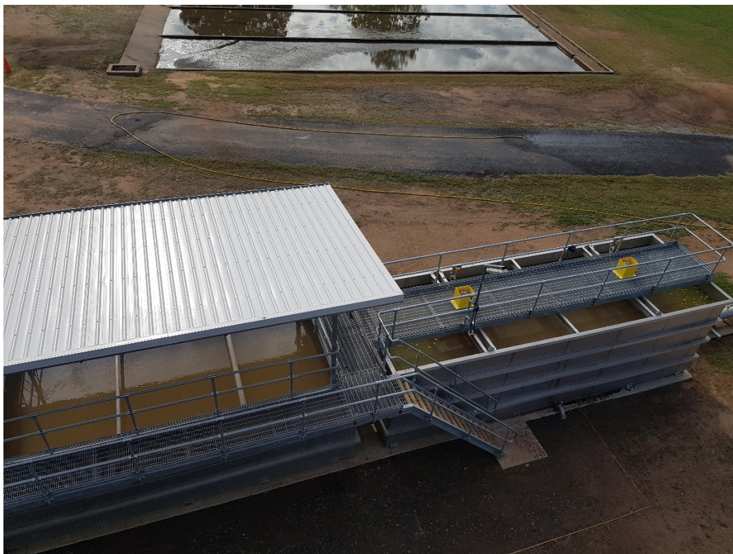
Figure 0-5: DAF Unit at Dysart WTP
