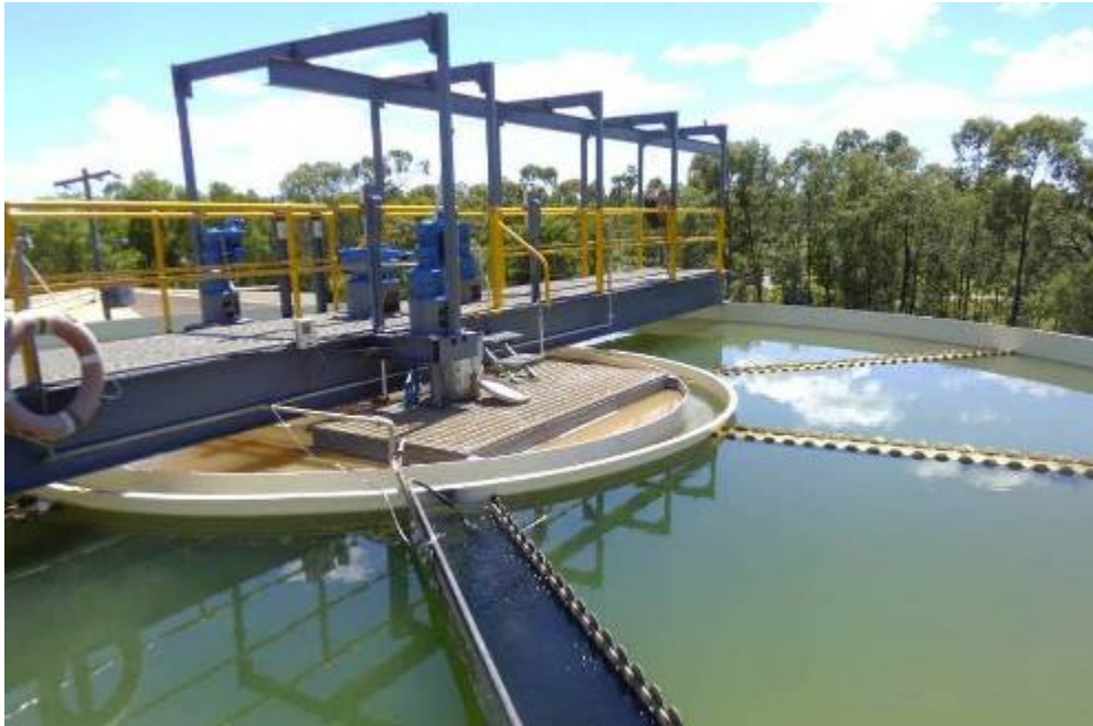
Figure 0-5: Clarifier with Central Flocculation Chamber
