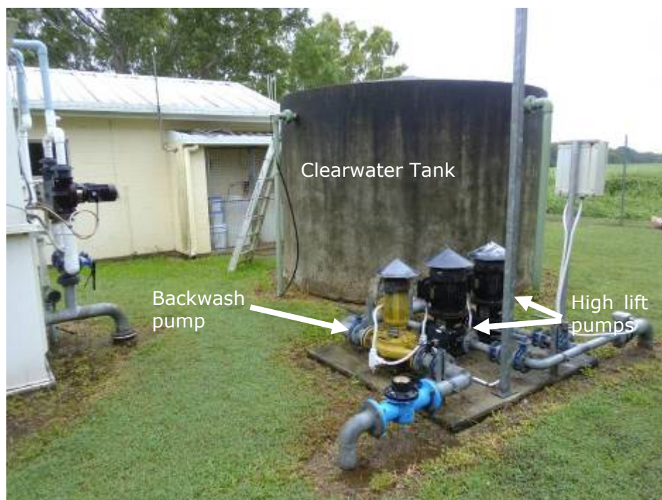
Figure 0-7: Clearwater Tank, High Lift Pumps and Backwash Pump
