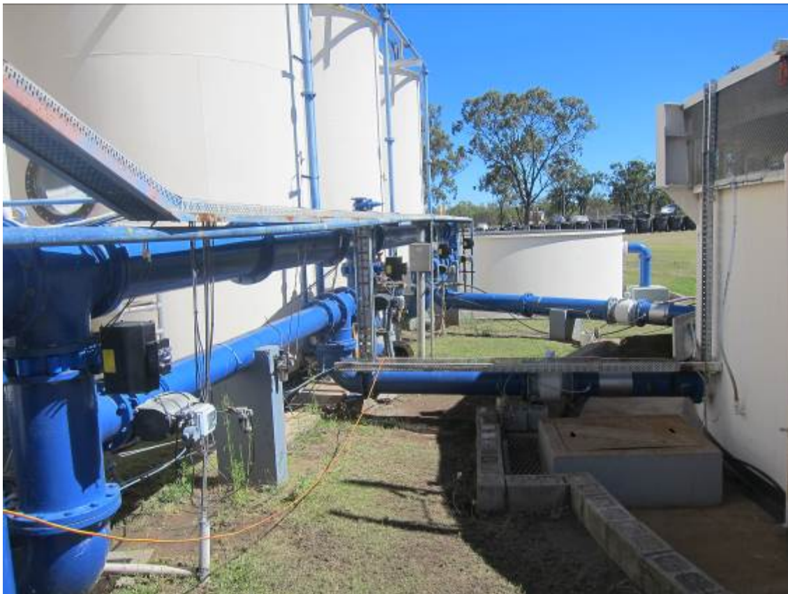
Figure 0-9: Filtered Water Manifold to Clearwater Tank
