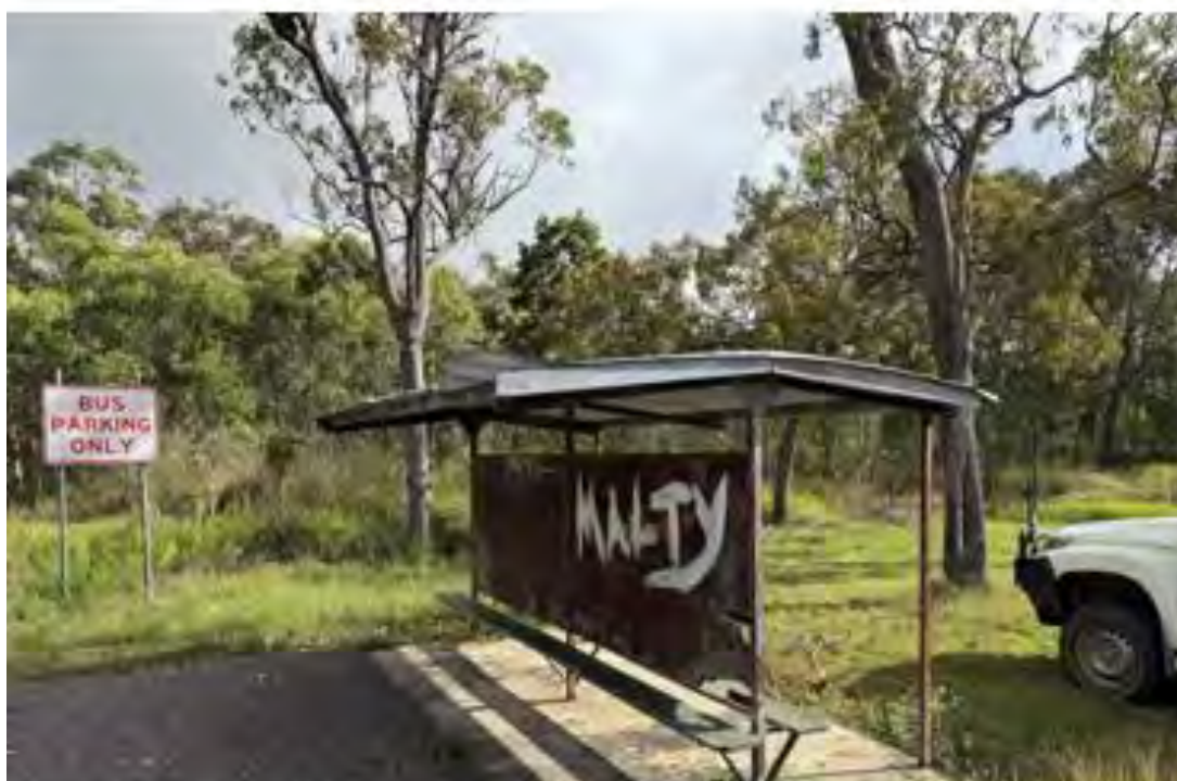
Image 2 – Ilbilbie bus shelter – this image illustrates deteriorated condition of the structure and damage to roofing sheets caused by vehicle collision.
