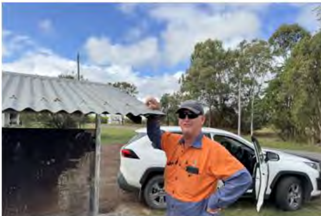
Image 1 - Carmila bus shelter – this image illustrates shelter height, possessing serious risk to the users due to no capping and sharp edging of the roof sheeting.
