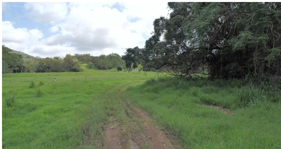
Figure 3: Road condition as at 21 January 2026
