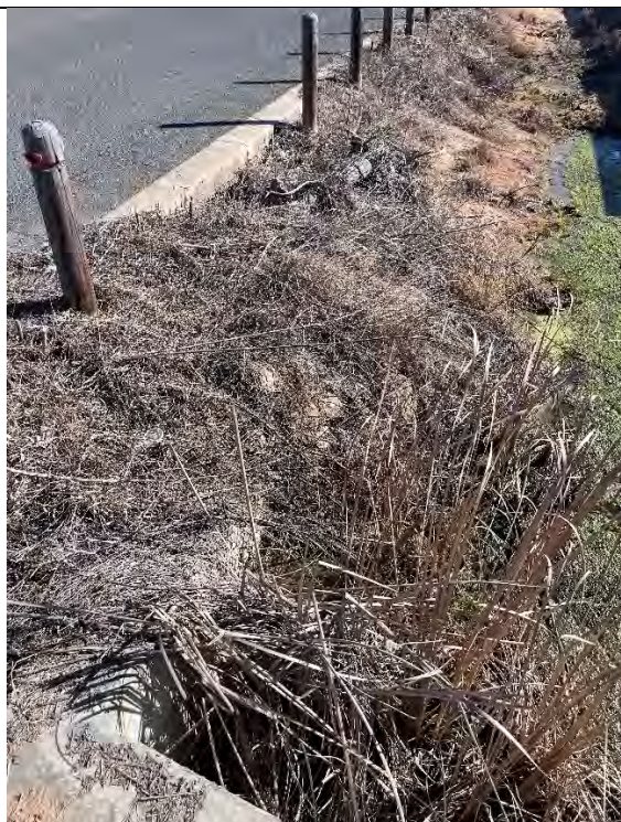
Erosion towards the road has de-stabilised the footings for the reflective marker posts
