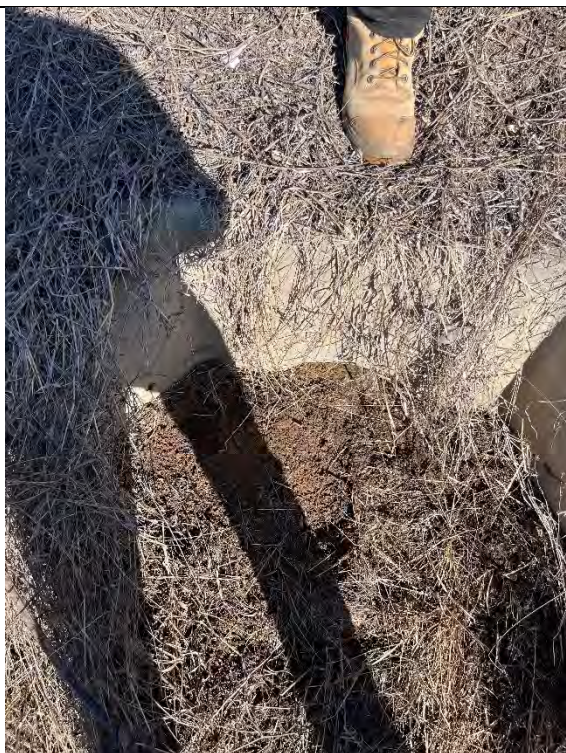
Sediment filled outlet that drains into the open channel drain – drain is fed by field inlets.
