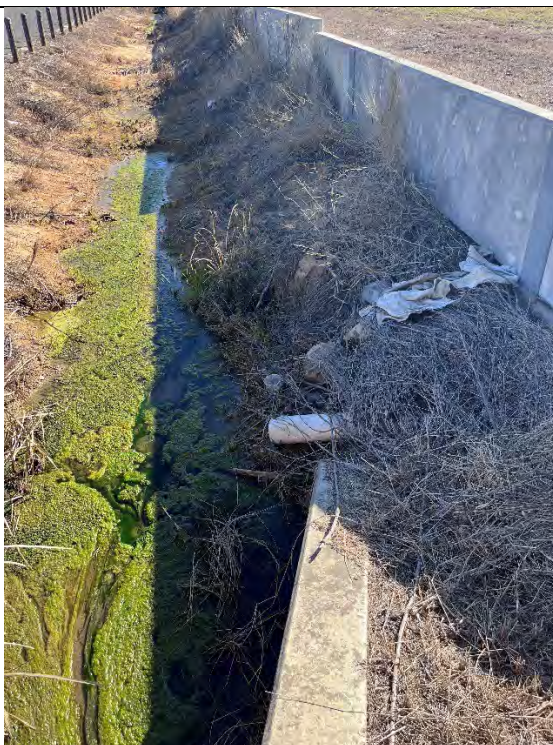
Water ponding and erosion of channel sides
