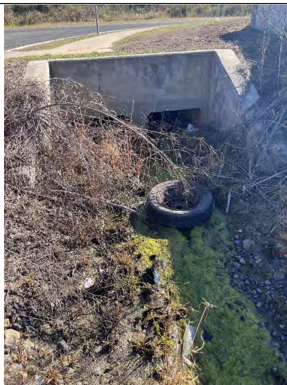
Blockage and buildup at Western channel inlet
