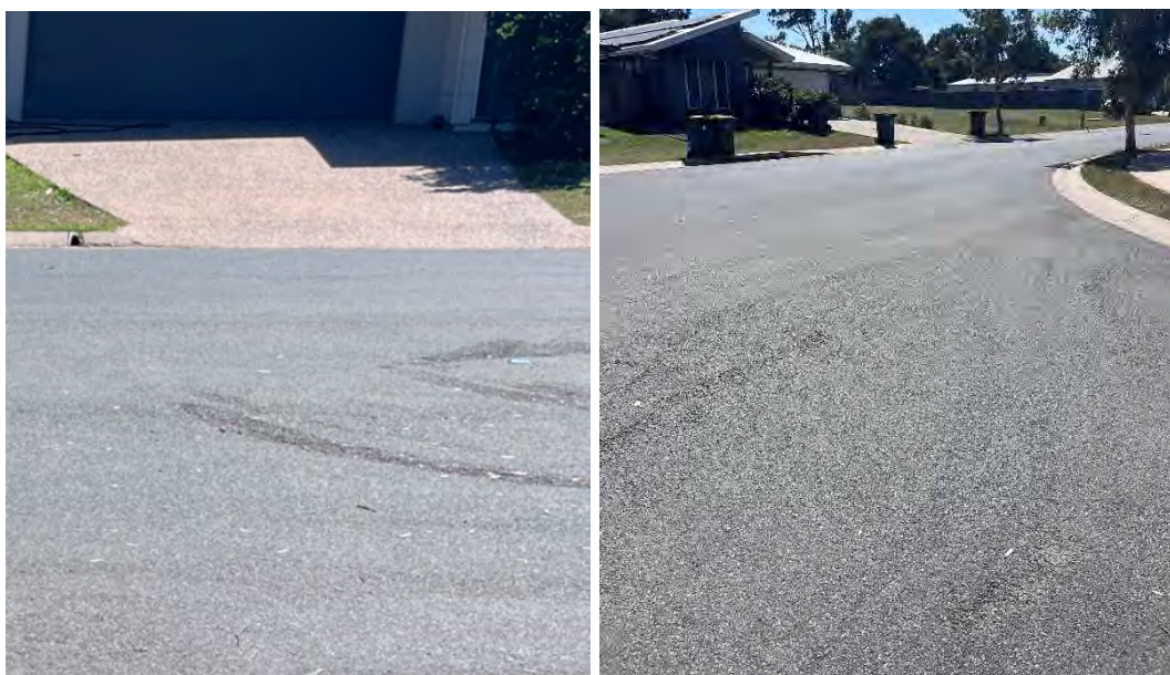
Figure 1 – Rosella Court Screwing Damage
