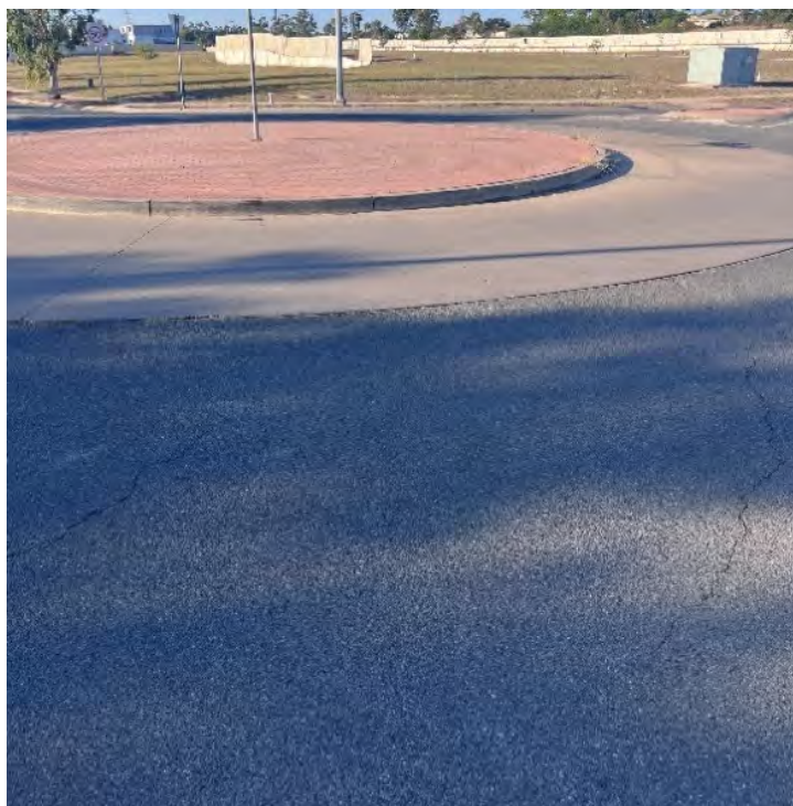
Figure 7 - Asphalt Cracking at Mills Ave. Roundabout
