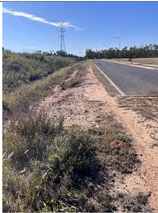
Vegetation growth in inlet drain
