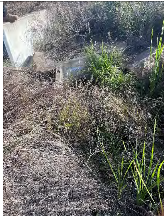
Main culvert blocked by vegetation
