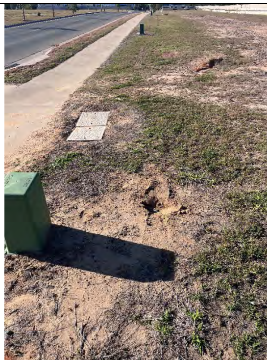
Complete sediment cover of field inlet pit
