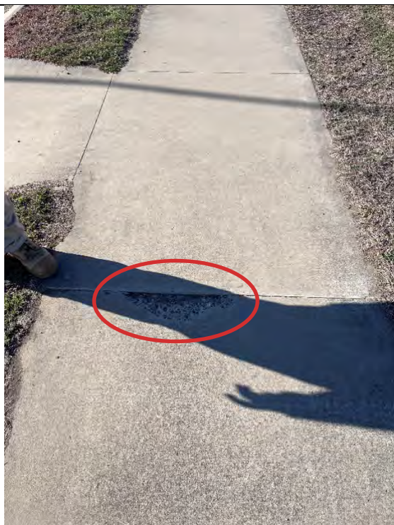
61 Shaw Street Minor Spalling at expansion joint
