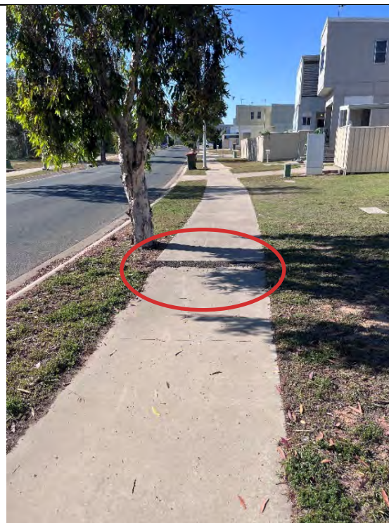
155 Utah Drive Concrete height + difference filled with asphalt
