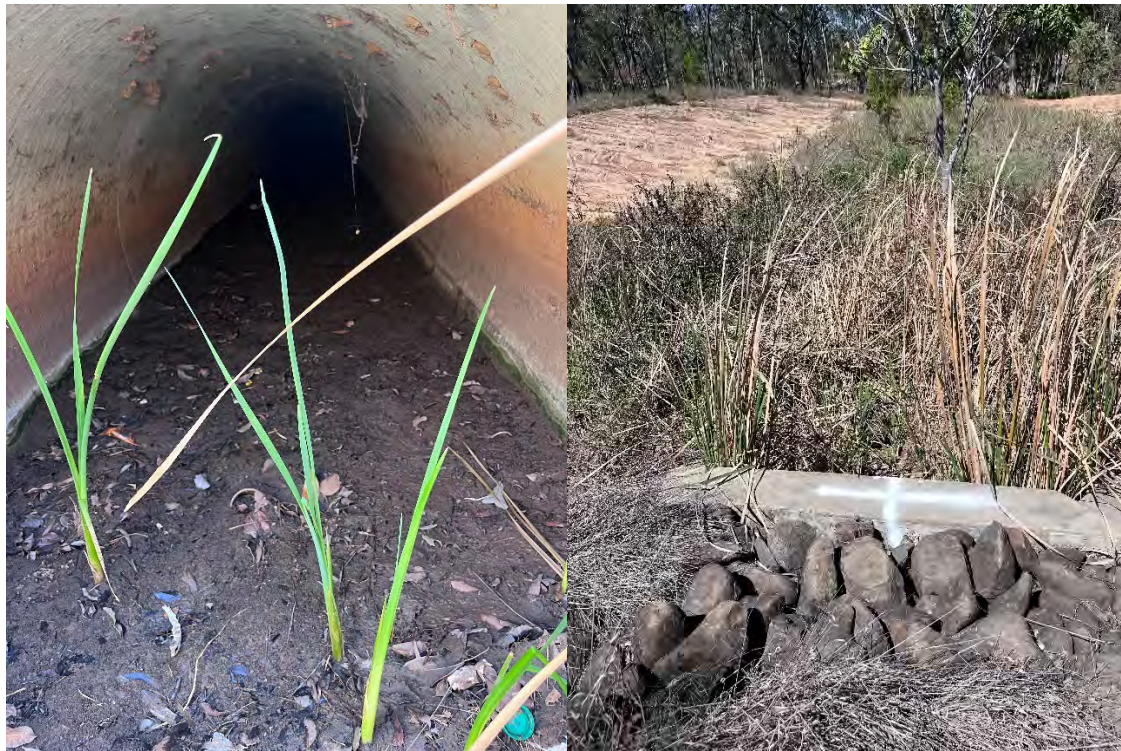
Figure 13 - Stormwater Outlet Buildup
