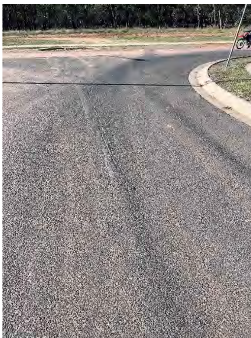
Figure 8 - Asphalt Cracking at Gardner Street Northern Int.
