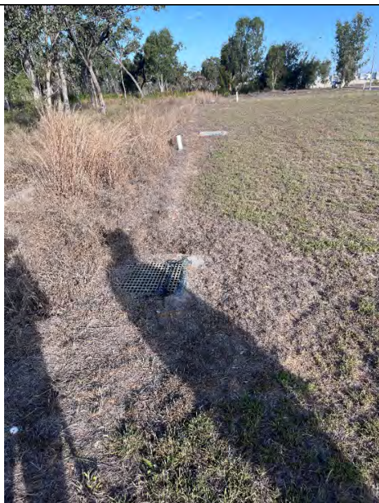
Partial sediment cover of field inlet pit
