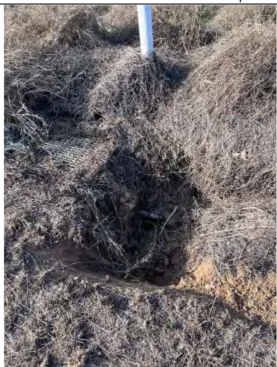
Settlement around field inlet
