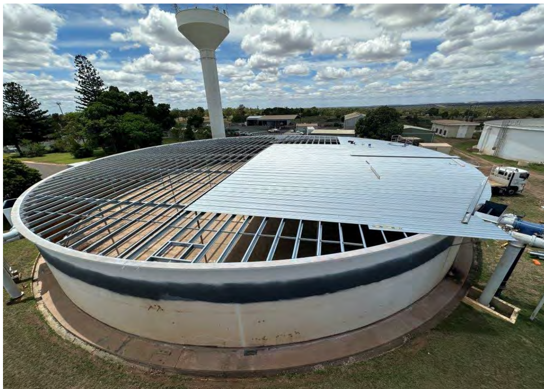
Image 1: Moranbah Water Treatment Plant Roof Replacement – Roof sheeting installation
