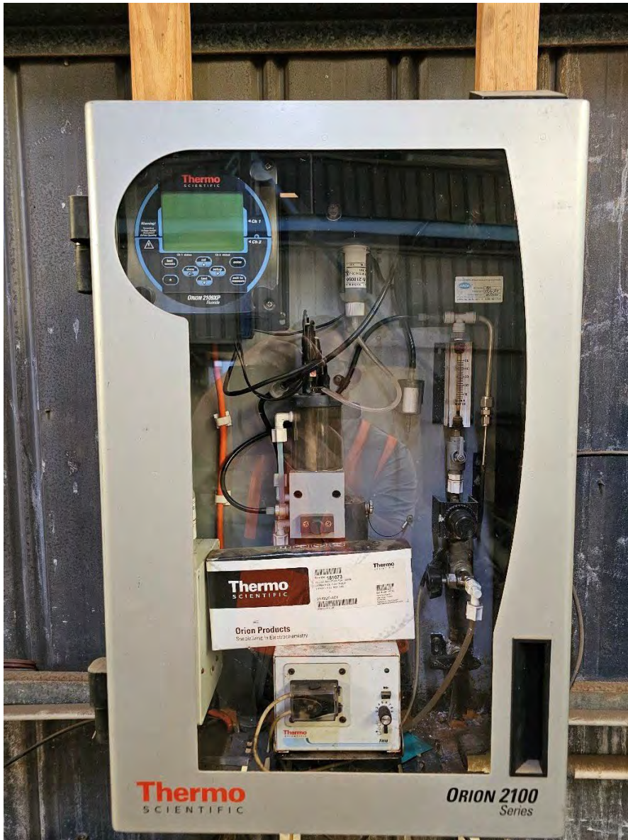
Photo 5: Moranbah WTP Fluoride Analyser (not currently operating)
