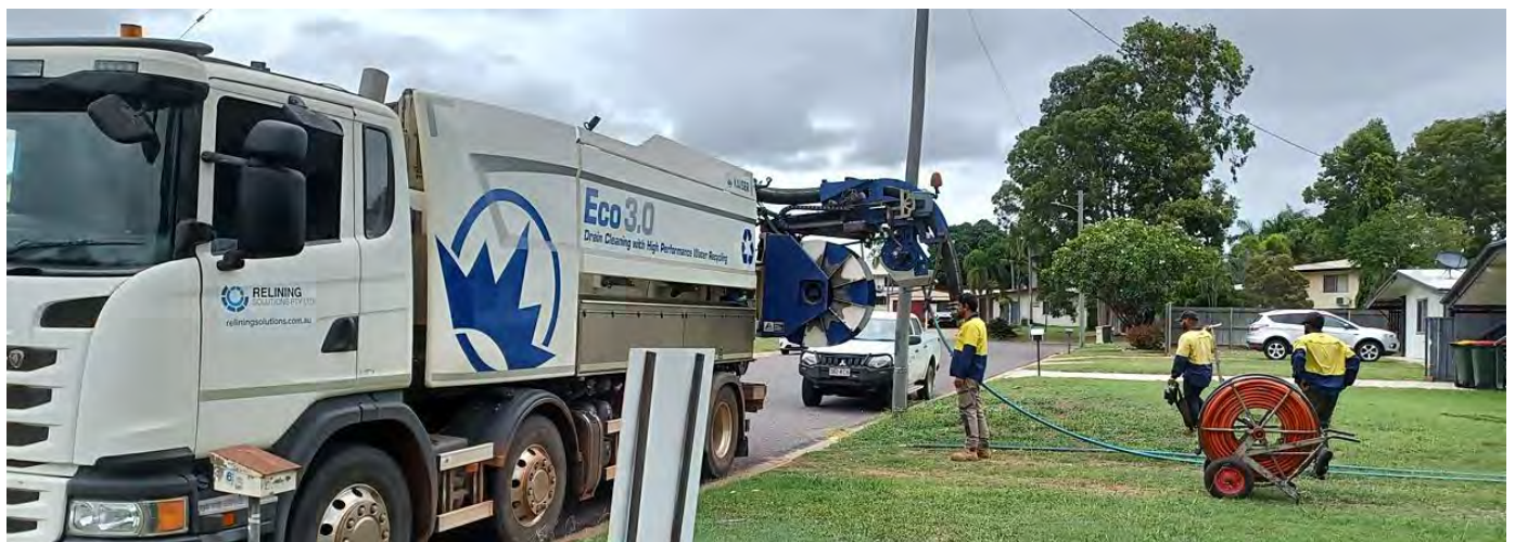
Image 5: COPR Sewer Relining – CCTV Camering on Barcoo Drive Moranbah in Progress
