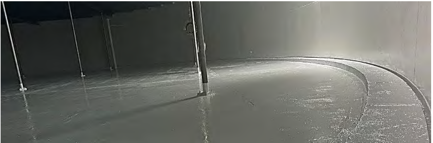
Image 1: Moranbah Water Treatment Plant Roof Replacement – Floor and Wall Epoxy Complete
