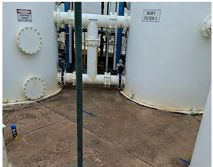
Image 5: Moranbah Water Treatment Plant Drinking Water Compliance – Marking Out Turbidity Analyser Locations
