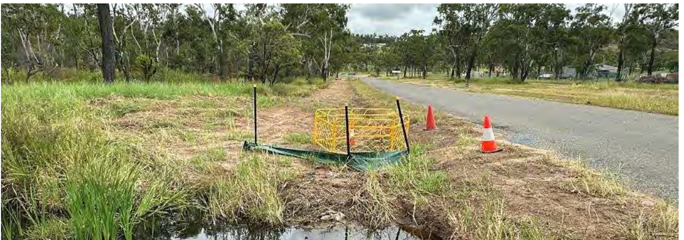
Image 4: Middlemount Water Network Augmentation – Water Main Roadside Alignment being cleared
