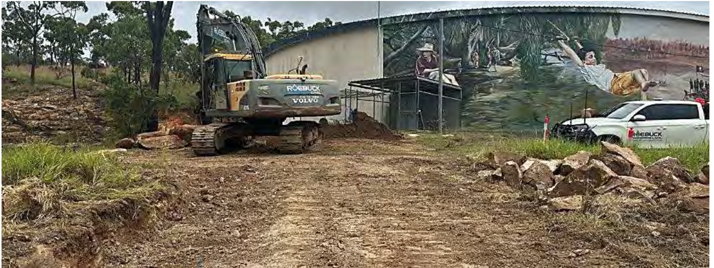
Image 3: Middlemount Water Network Augmentation – Water Main Alignment near Reservoir being cleared
