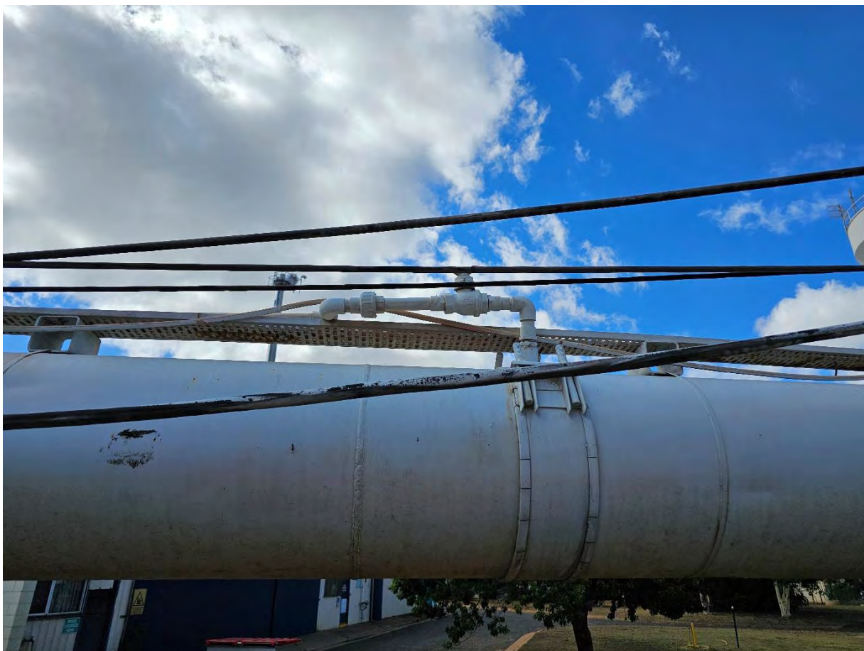
Photo 29: Moranbah WTP Bobby Plant Fluoride Injection Point – Compliant with Code of Practice Item 3.7.1
