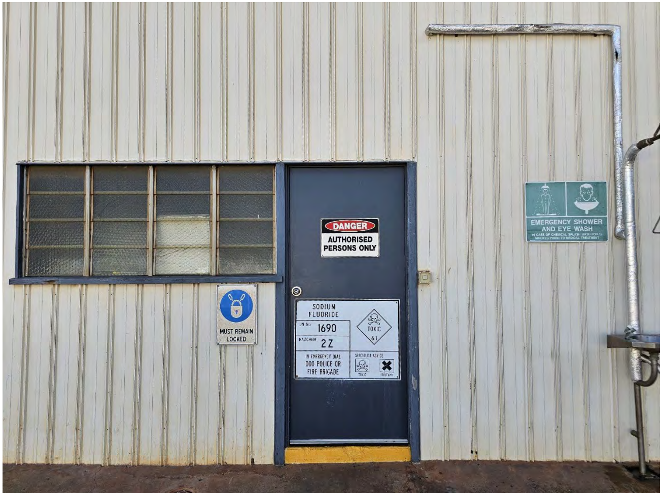
Photo 1: Moranbah WTP Fluoride Batching Rom
