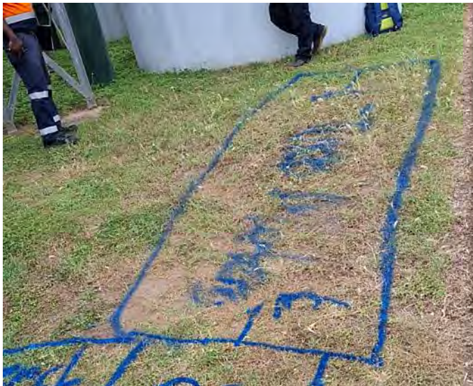
Image 5: Moranbah Water Treatment Plant Drinking Water Compliance – Marking Out Turbidity Analyser Locations
