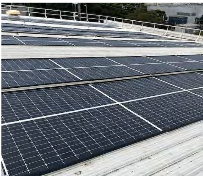
Figure 7. Light weight panels installed on the Pfizer building in Melbourne (courtesy Integrated Energy Solutions 18 )
