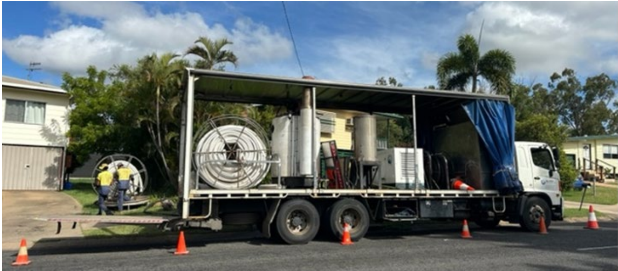
Image 4: Sewer Relining in progress on McCool Street, Moranbah
