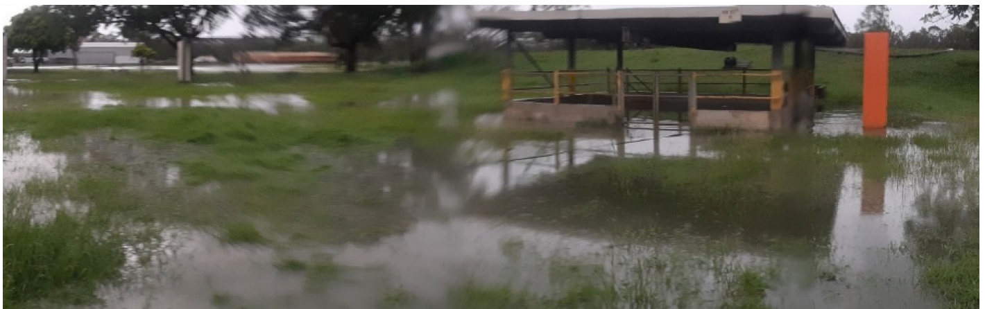
Image 2: Standing water at MMT WTP
