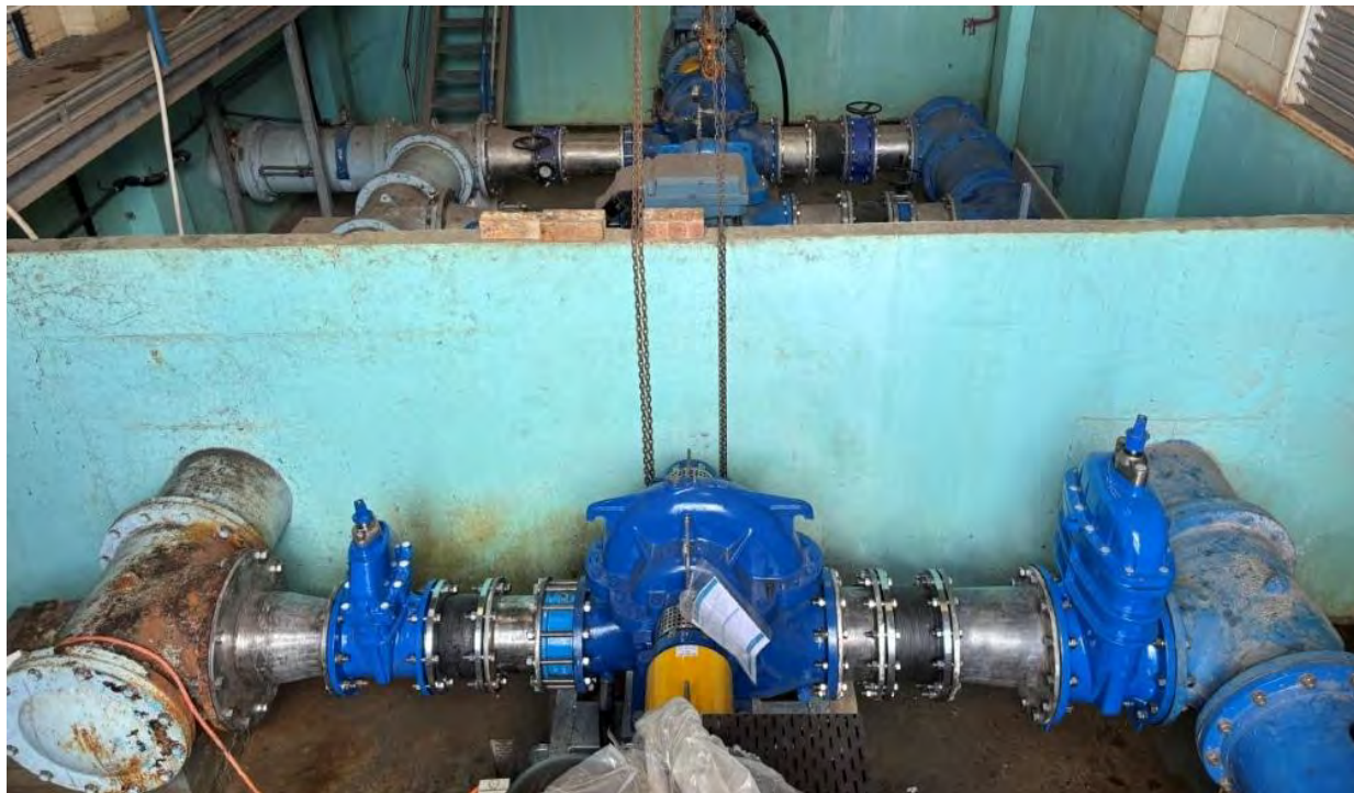
Image 3: MBH WTP West & East High Lift Pumps - East Tower Pump Station new diesel pump & valve installation
