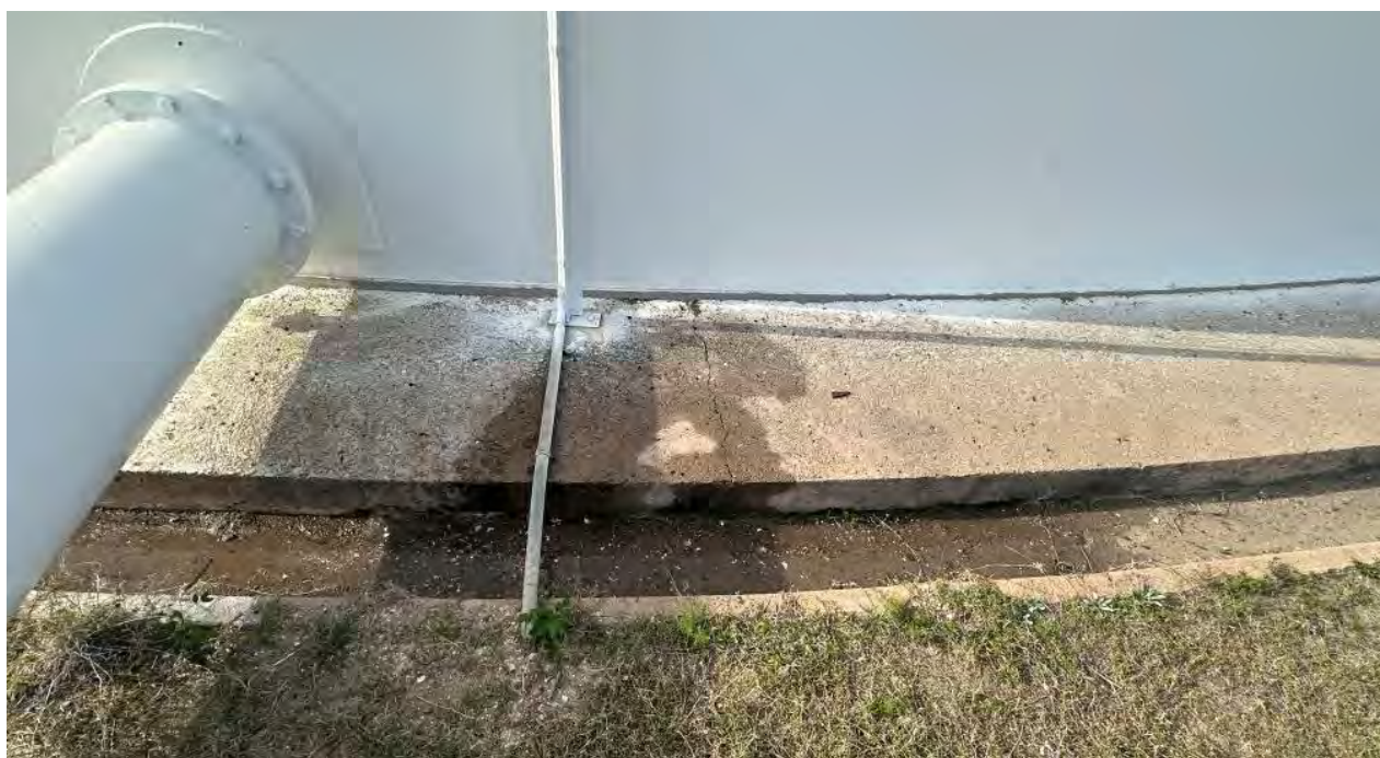
Image 4: MBH WTP Roof Replacement – remaining leak on join between tank wall & concrete floor on outlet of 5.7ML Reservoir
