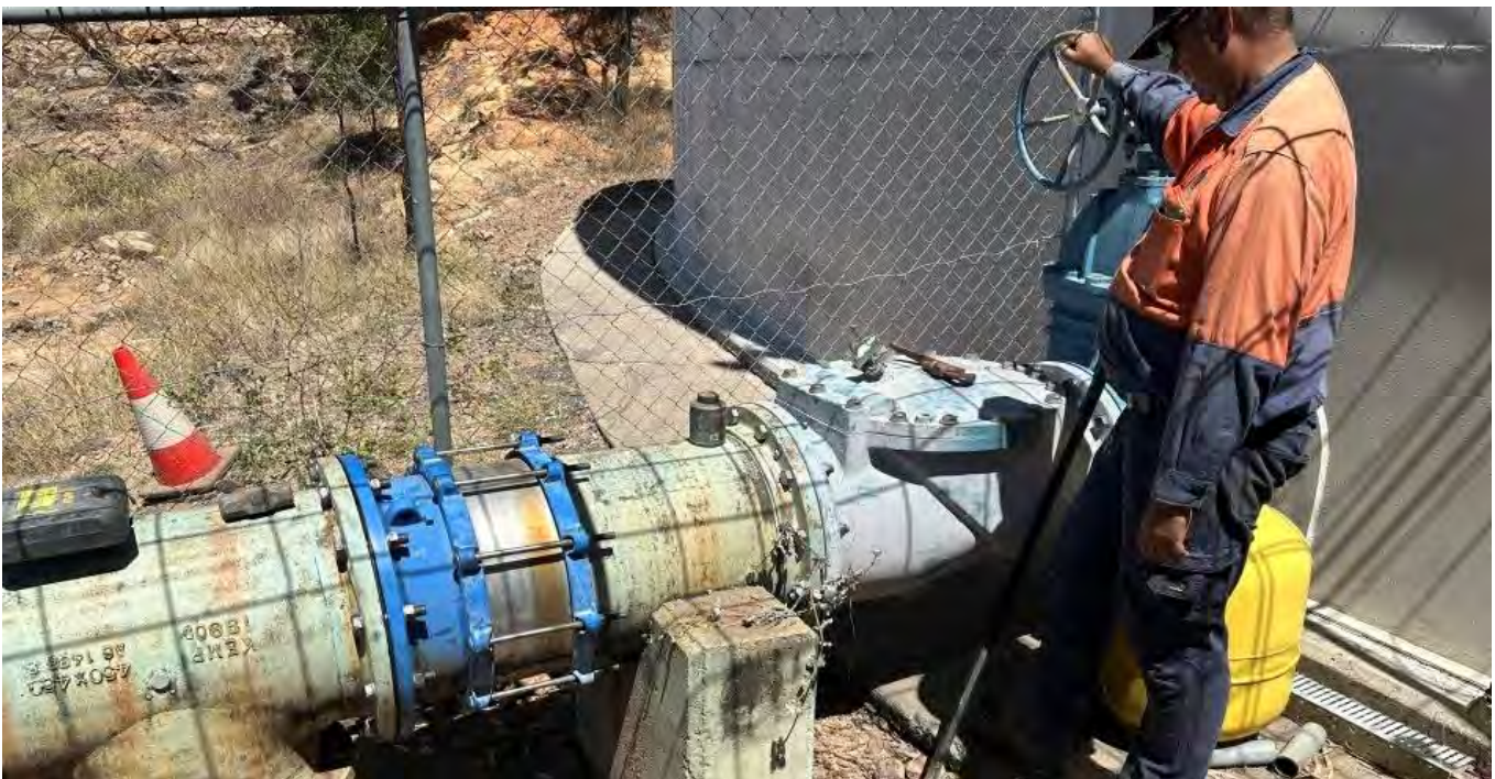
Image 1: MMT WN Augmentation – opening valve on inlet line of 8ML Reservoir
