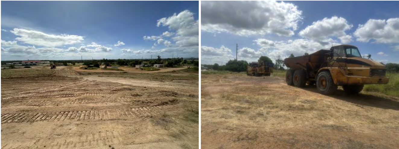
Image 3: MBH Rectification of Landfill Cell – Stripping & stockpiling of materials
