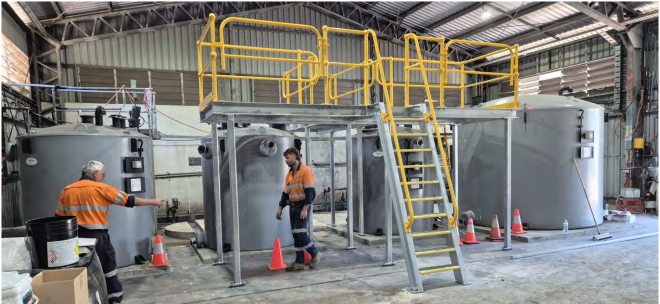
Image 2: CLM WTP Filter Media and Plant Modernisation – Installation of Walkways
