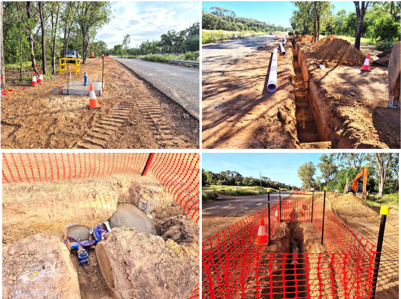
Image 1: MBH Recycled Water Network - Irrigation pipeline installation along Sarchedon Drive
