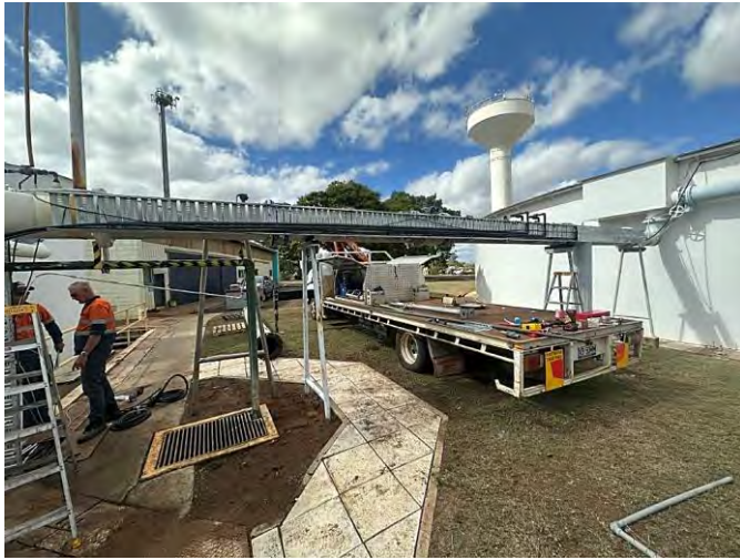
Image 3: MBH WTP Install Baby Plant flow meter
