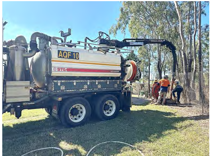
Image 4: CORP Sewer Relining
