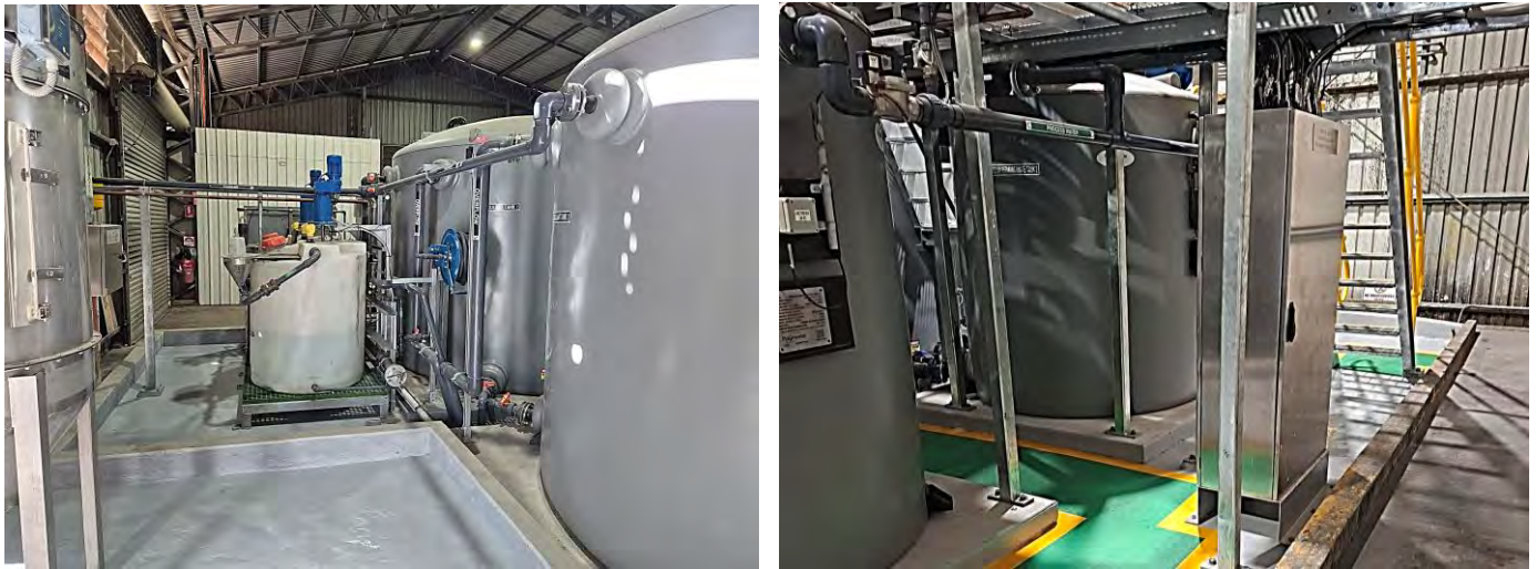
Image 1: CLM WTP Modernisation – chemical dosing upgrade
