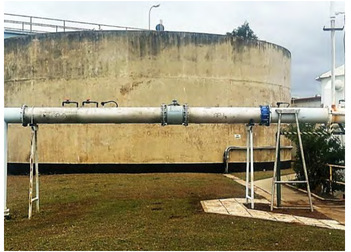
Image 3: MBH WTP Install Baby Plant flow meter
