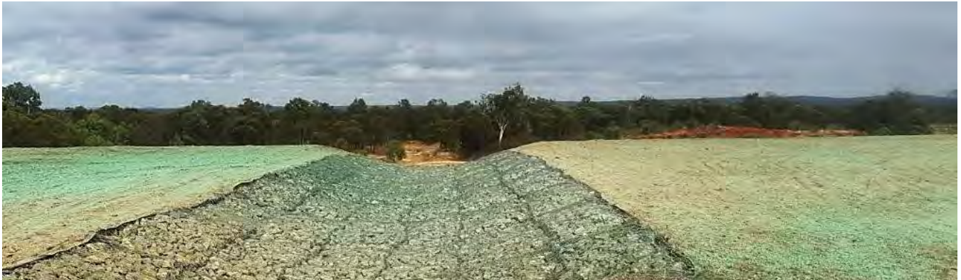
Image 6: Moranbah Cell 0 Landfill Rectification
