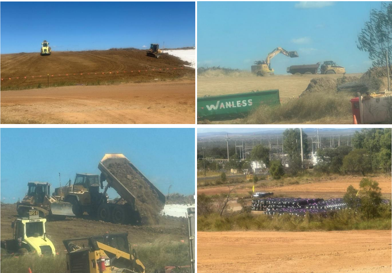
Image 3: MBH Rectification of Landfill Cell – GCL stockpiling & preparation
