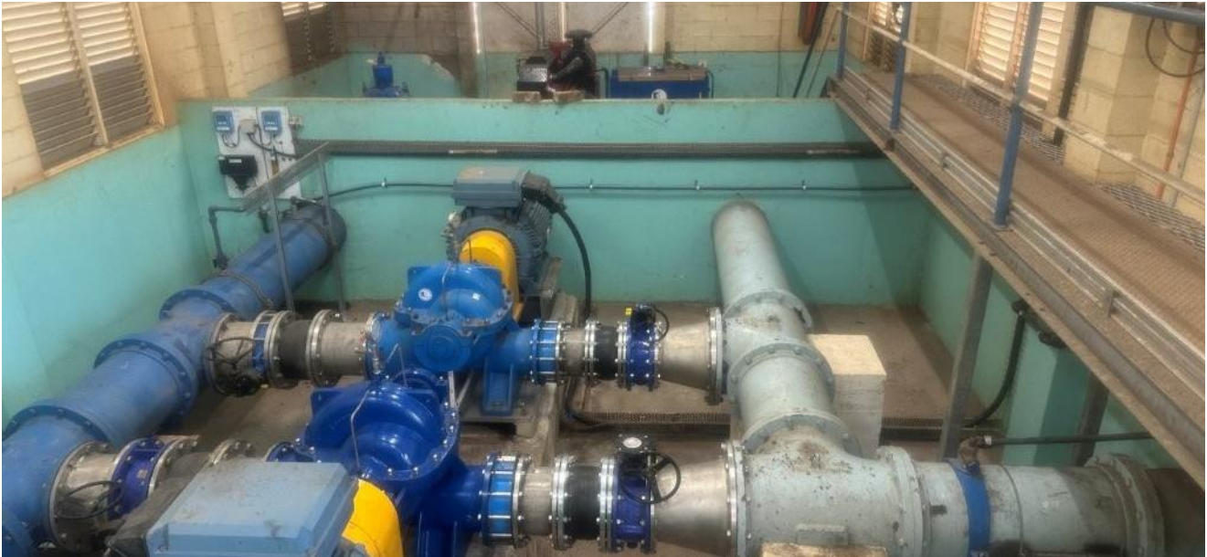
Image 2: MBH Pump Station 2 – installation of pumps, valves and pipework
