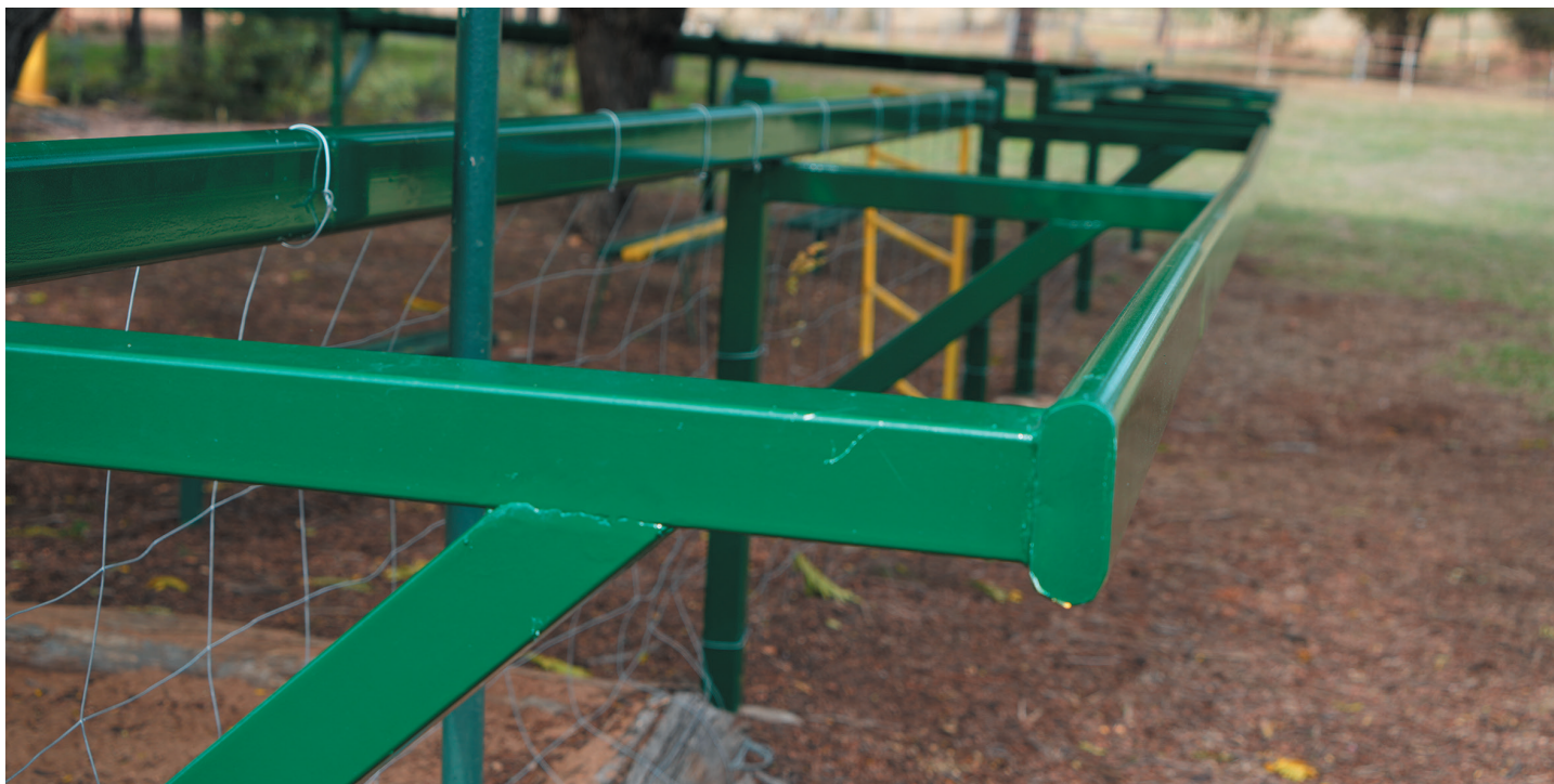
These rails were manufactured and installed by Clermont Work Camp prisoners
