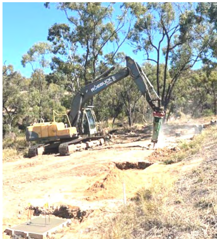
Image 1: MMT WN Augmentation – installing standard bases & rock removal
