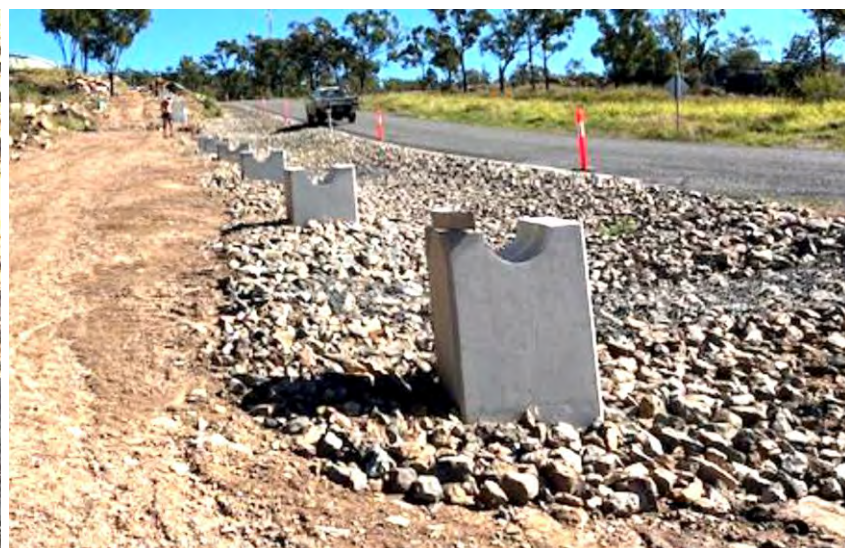
Image 2: MMT WN Augmentation - Installing piers
