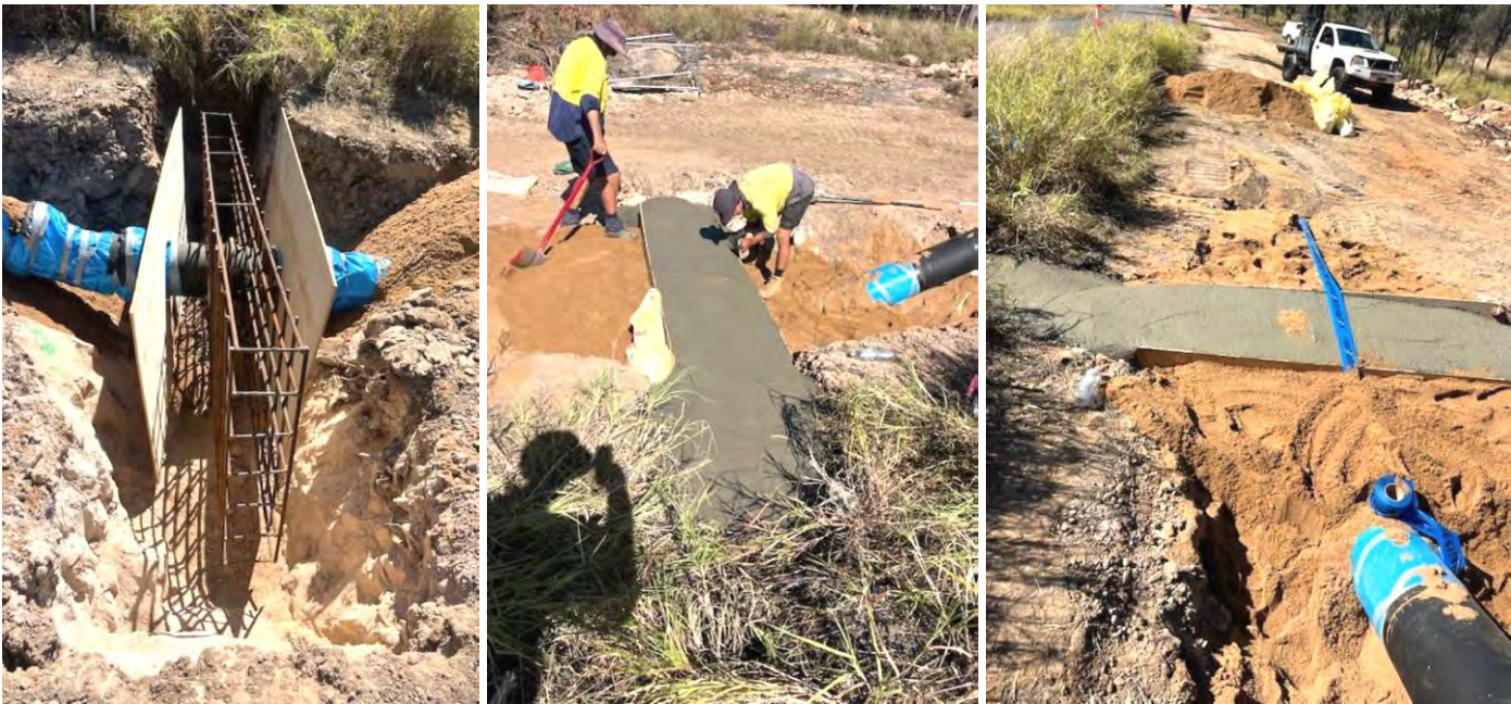
Image 3: MMT WN Augmentation - Install inline thrust blocks
