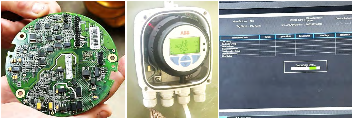
Image 4: MMT Sewer Pump Station 01 – Remediation of ABB Flow Meter
