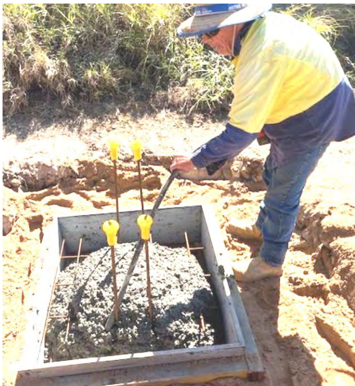
Image 1: MMT WN Augmentation – installing standard bases & rock removal
