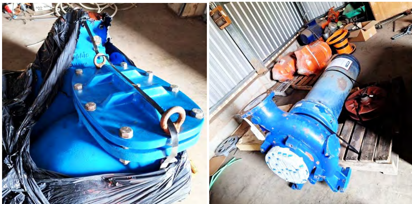
Image 6: Moranbah Sewer Pump Station 01 – Pump & NRV replacement
