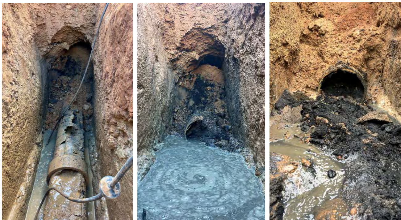
Image 4: CORP Sewer Relining 2025 – collapsed pipes in Flight Street, MBH
