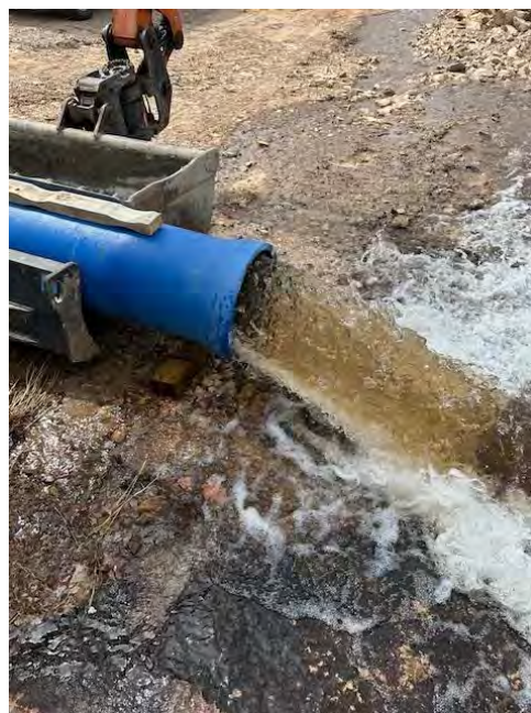
Image 2: MMT WN Augmentation – flushing pipe from Water Treatment Plant to start of above ground section
