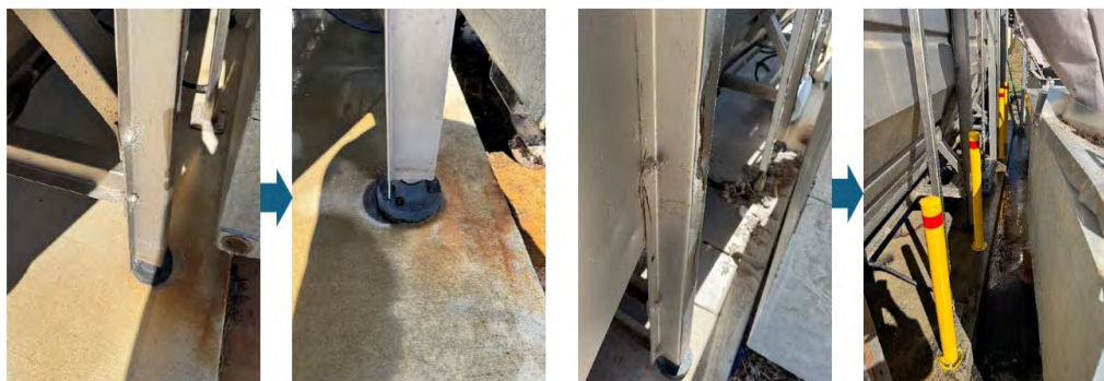
Figure 1 Example of Inlet Screen Proactive Maintenance (Left: Equipment shift to secure location, Right: Install structural protection)
