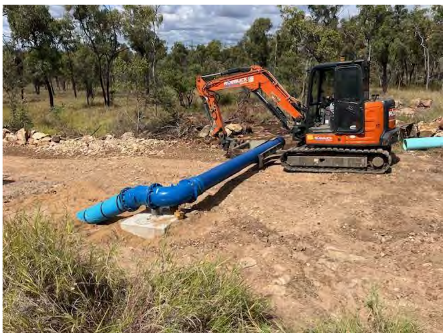
Image 2: MMT WN Augmentation – flushing pipe from Water Treatment Plant to start of above ground section
