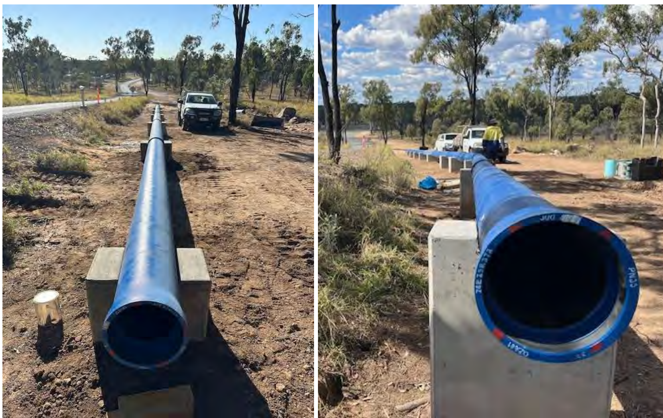
Image 3: MMT WN Augmentation – installing pipe above ground
