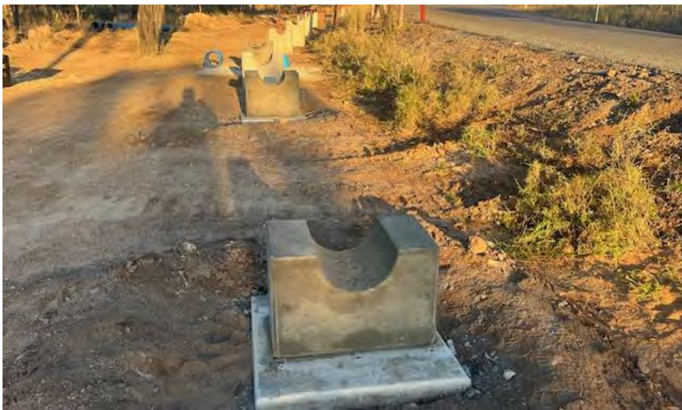
Image 1: MMT WN Augmentation – installing piers
