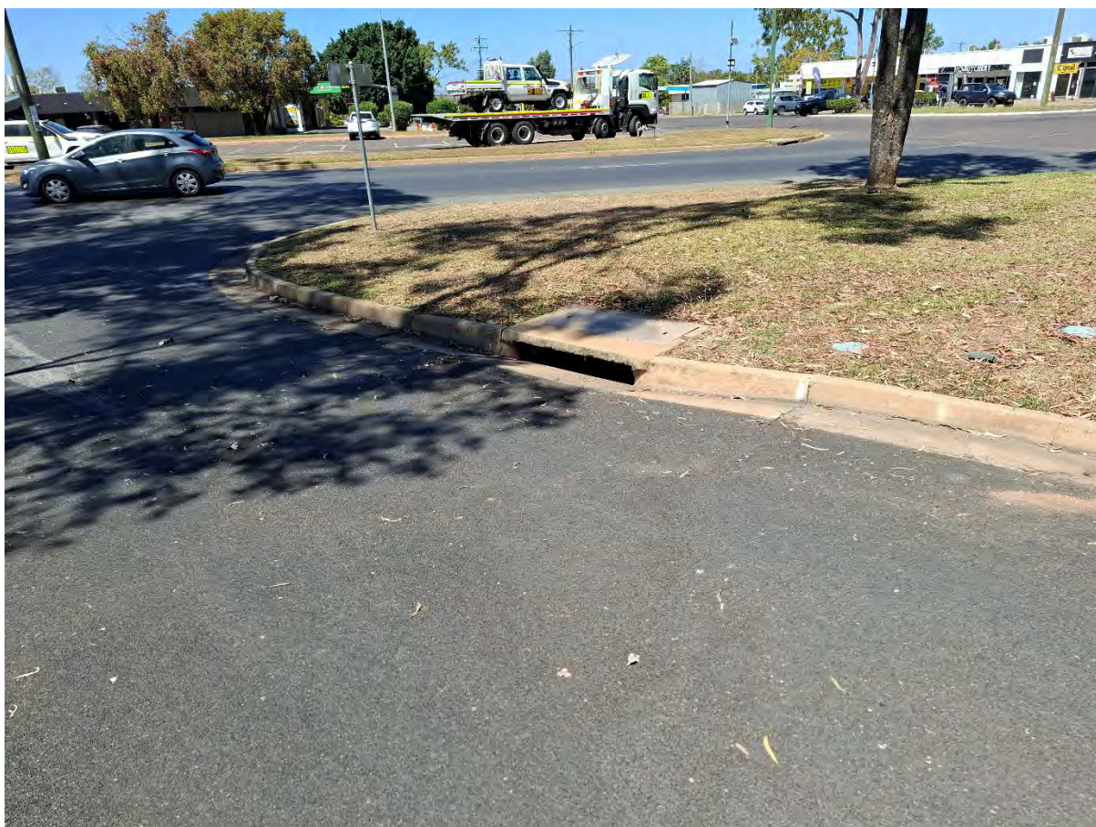
Storm water drain to consider screening to prevent access
