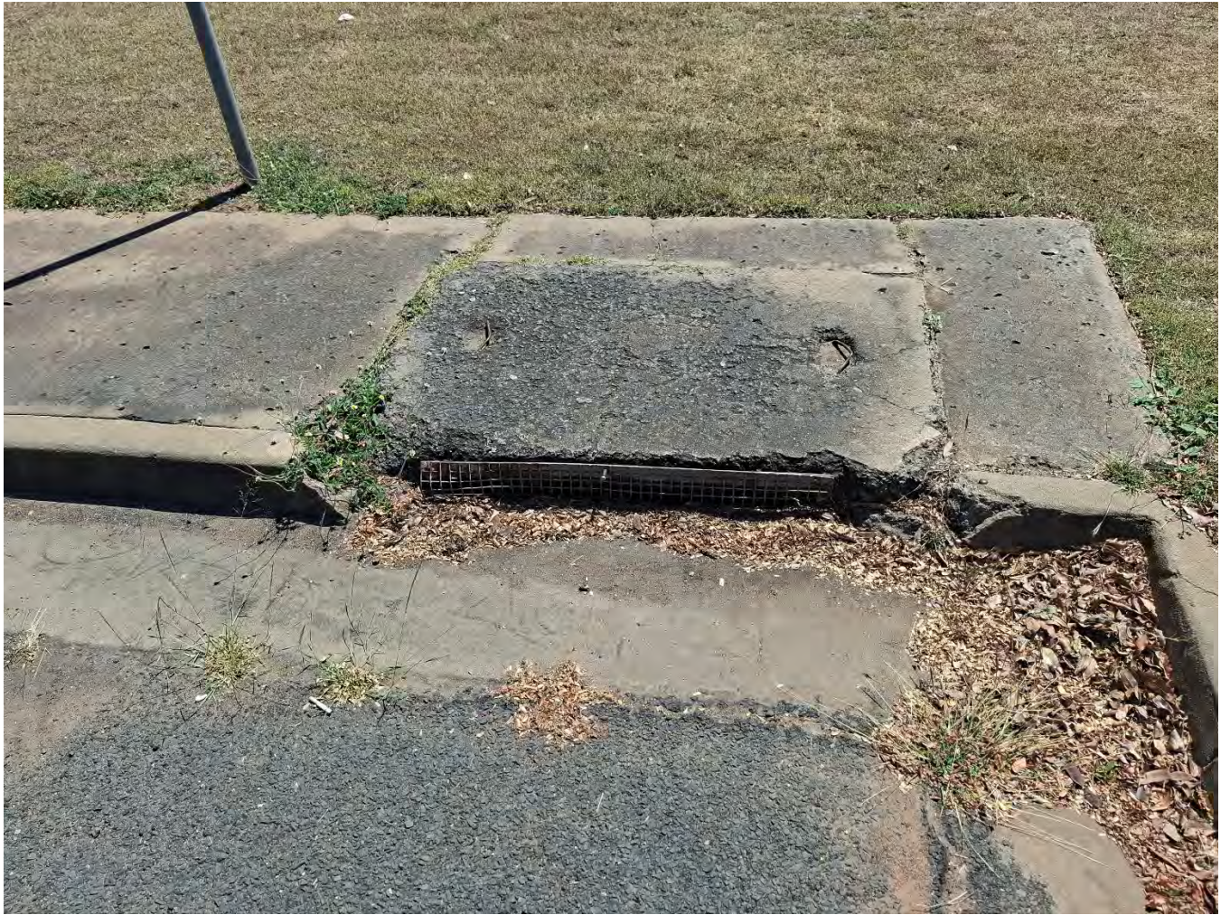
Repair to gross pollutant trap to prevent access
