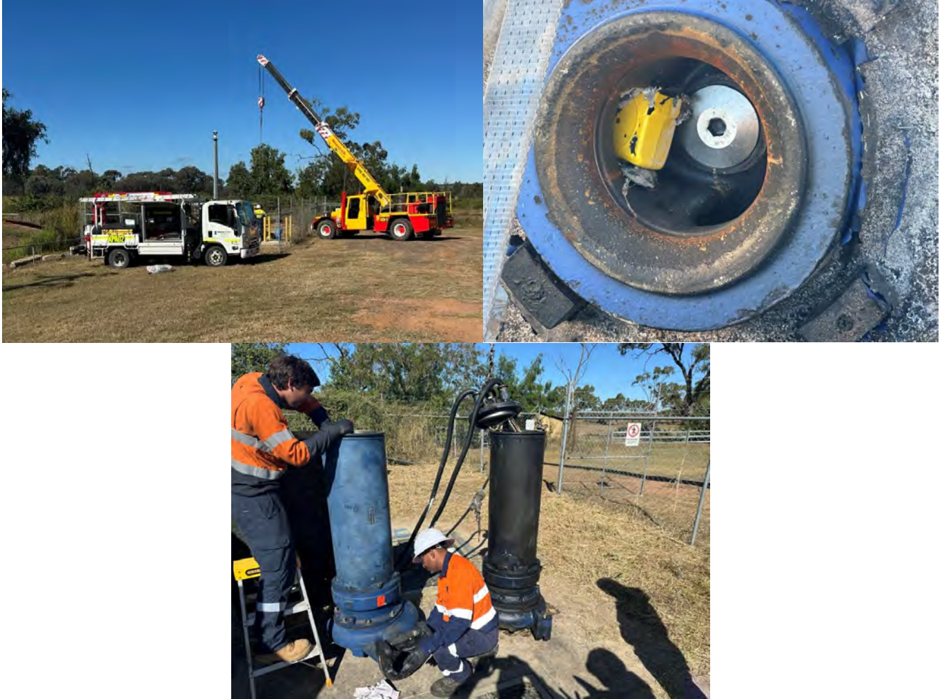
Image 4: Moranbah Pump Station 01 – Pump 1 replacement & transfer to Mackay to repair; tape jammed in impeller
