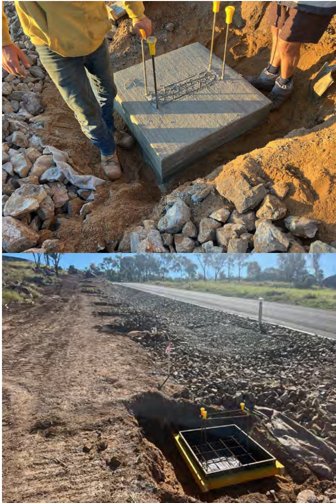
Image 3: Middlemount WN Augmentation – Plinths for above-ground water mains DICL
