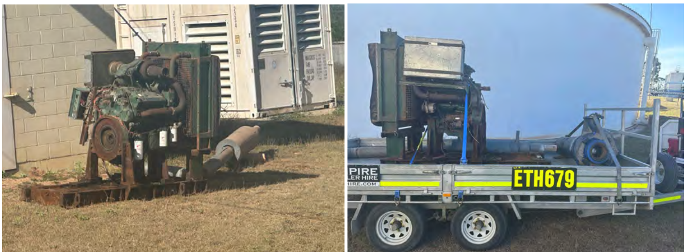
Image 5: Moranbah Water Treatment Plant East Tower Pump Station – diesel motor & pump removal
