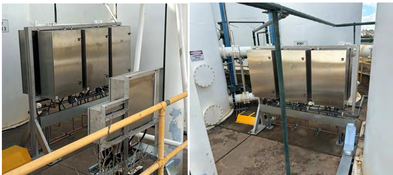
Image 2: Moranbah WTP Drinking Water Compliance –Installed Turbidity Analysers on Bobby Plant
