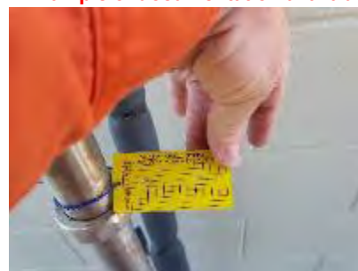
Example of testing and tagging of fire equipment
