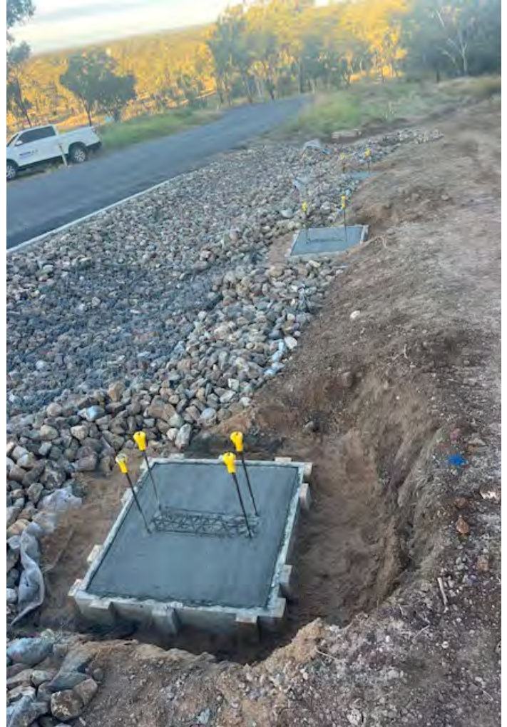
Image 3: Middlemount WN Augmentation – Plinths for above-ground water mains DICL
