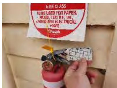
Demonstration of test and tag for firefighting equipment with signage
