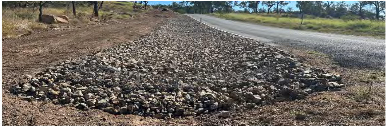
Image 4: Middlemount WN Augmentation – Drainage and Asphalt Complete
