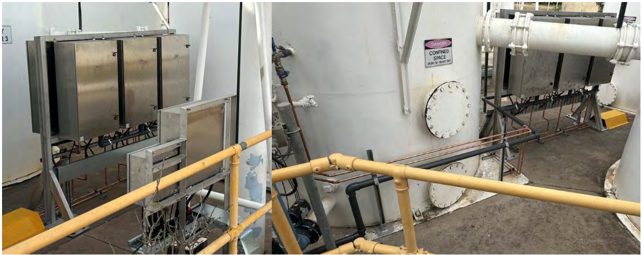
Image 3: Moranbah WTP Drinking Water Compliance –Installed Turbidity Analysers on Bobby Plant
