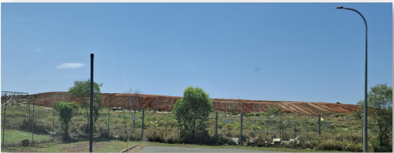
Figure 5 - Moranbah Landfill view from Thorpe Street, during the placement of interim capping on the Western batter of Cell 1 – October 2024
