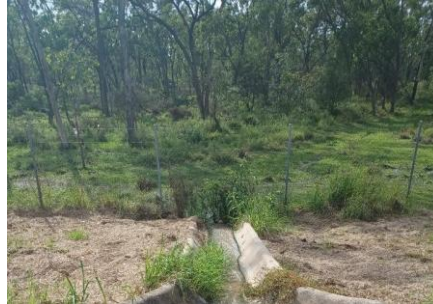
Middlemount Spillway Flow Area
