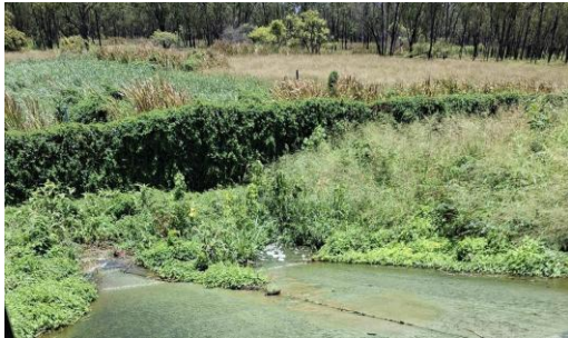
Moranbah Spillway Overtopping
