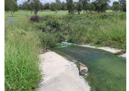
Dysart Spillway Flow Area
