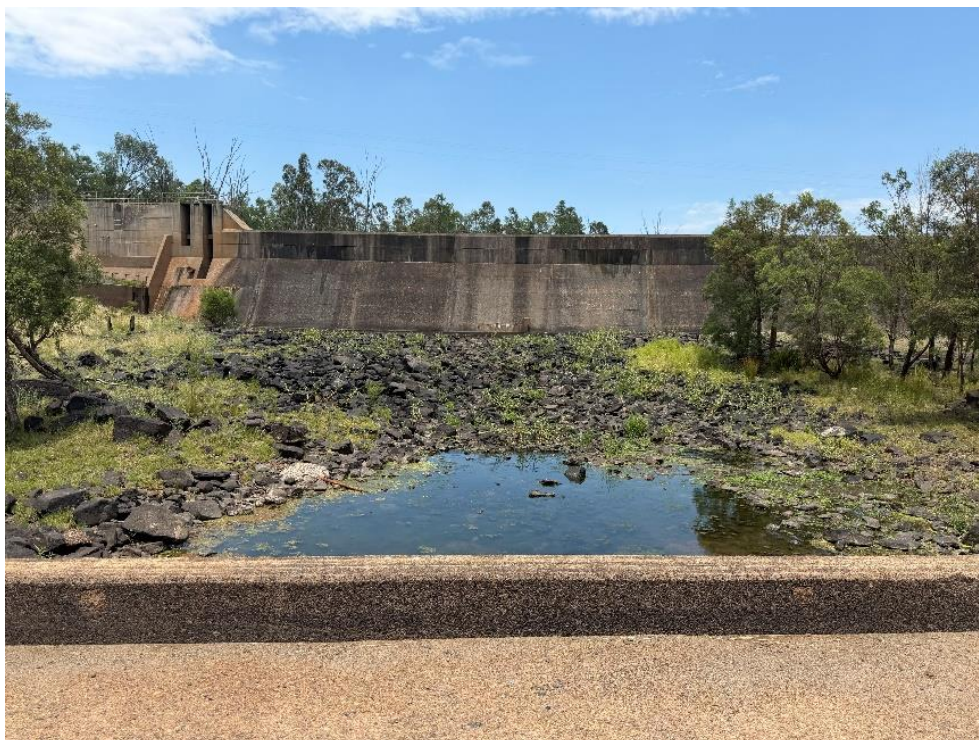
Figure 4-5 Bedford Weir (from downstream point of view)
