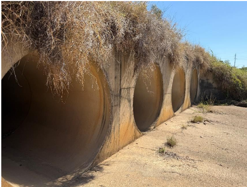
Figure 4-2 QLD TMR 4 x 1.8 m Diameter Circular Measured Culverts
