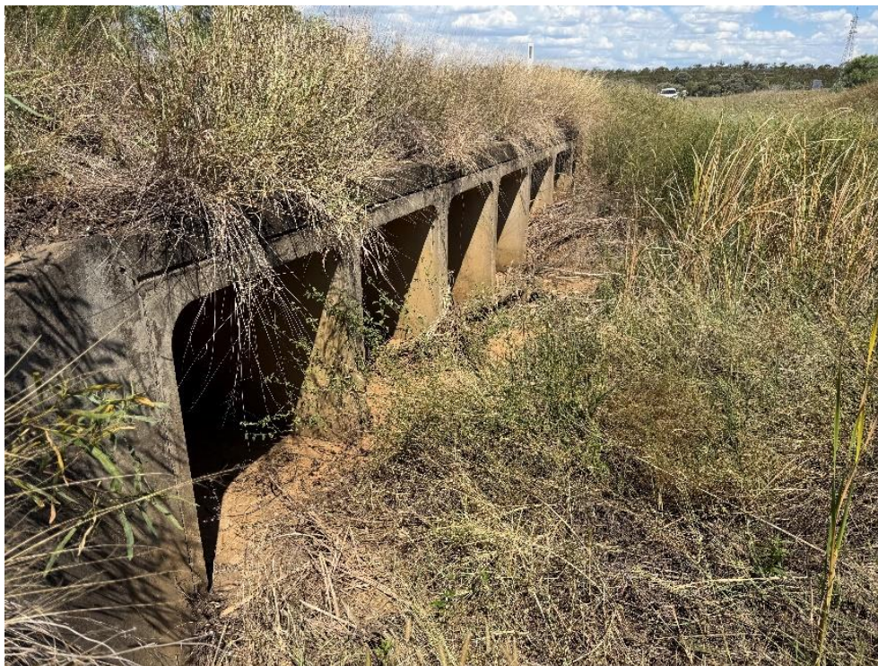
Figure 4-1 QLD TMR 8 x 1.2 m x 1.2 m Measured Box Culverts
