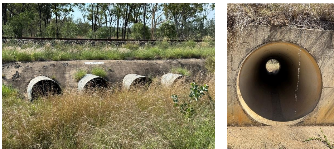
Figure 2-3 Hydraulic Structure Photographs Taken on Site
