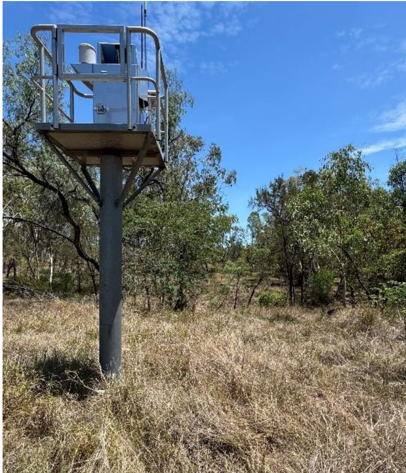
Figure 2-6 Sandy Creek Bridge TM Gauging Station
