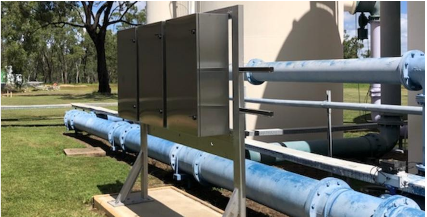
Image 4: Glenden WTP – Installation of Turbidity Analysers underway
