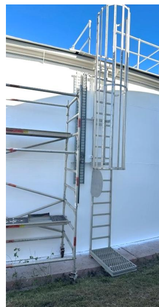
Image 1: Moranbah WTP Roof Replacement – Roof and Access Installation Complete
