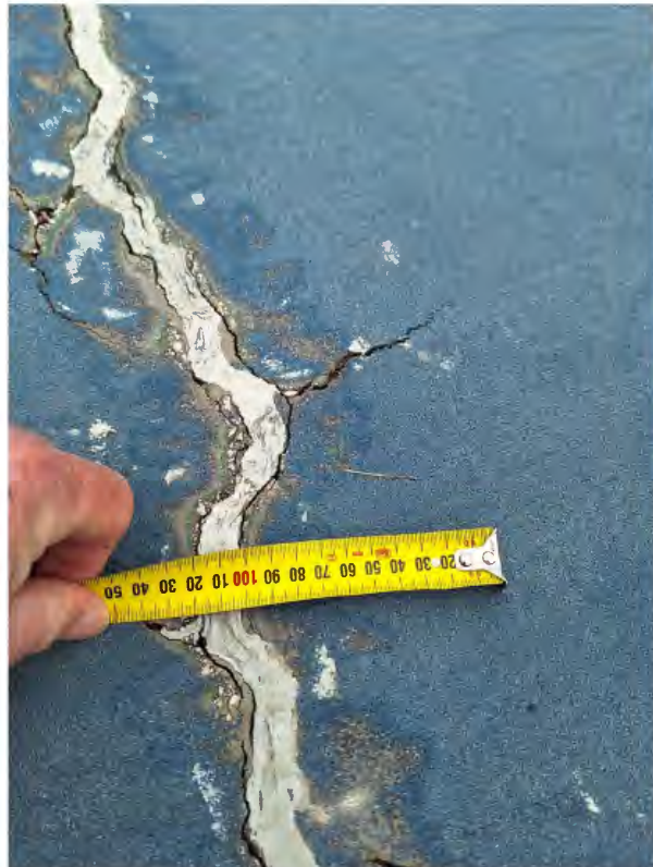
Images Demonstrating Width of Cracks in Tennis Court Surface
