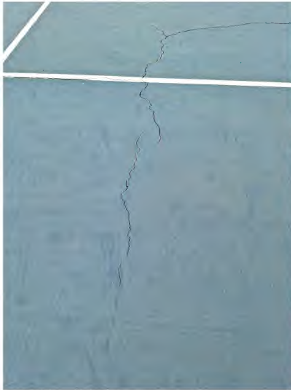
Images Demonstrating Width of Cracks in Tennis Court Surface
