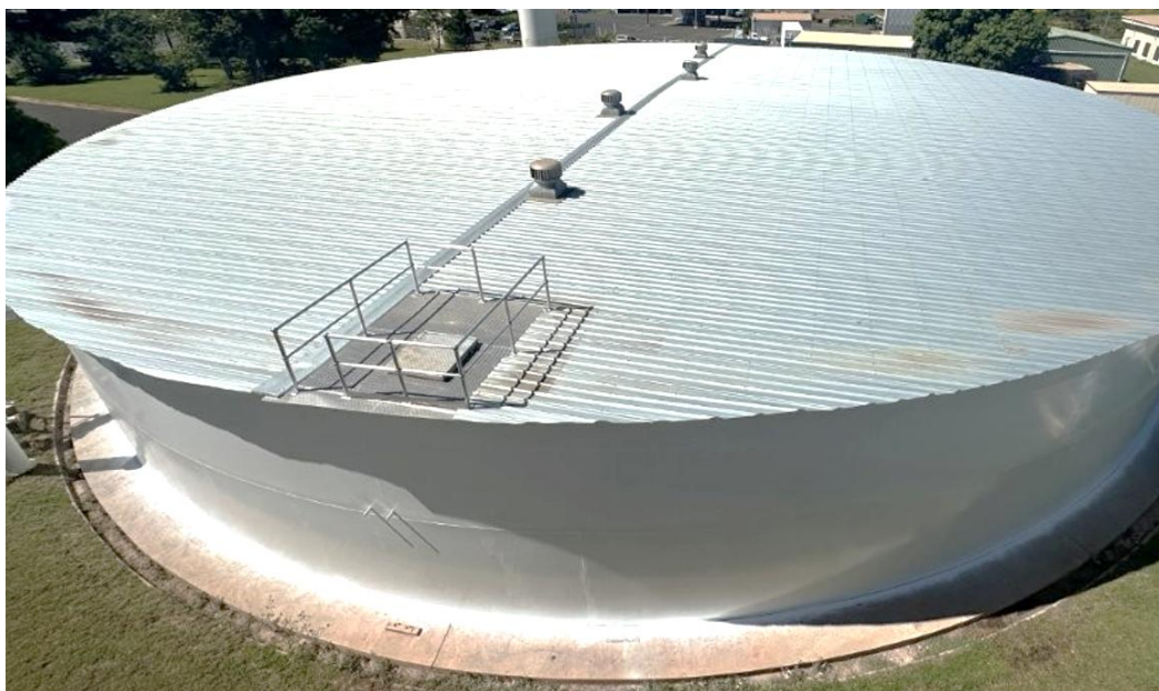
Image 1: Moranbah WTP Roof Replacement – Roof and Access Installation Complete
