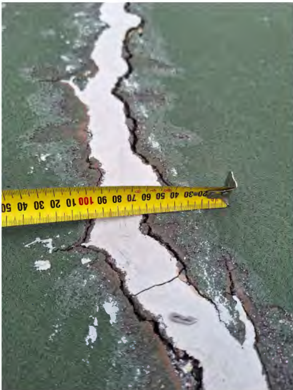
Images Demonstrating Width of Cracks in Tennis Court Surface
