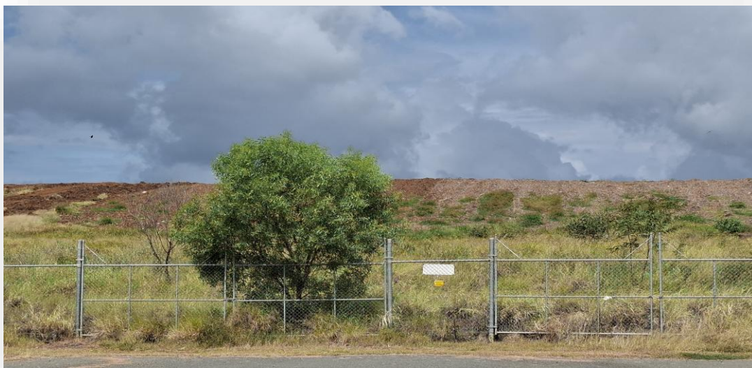
Figure 6 - Moranbah Landfill view from Thorpe Street, final cover with mulch in place with vegetation starting growth, along with all legacy litter removed on the Western batter of Cell 1 – March 2025
