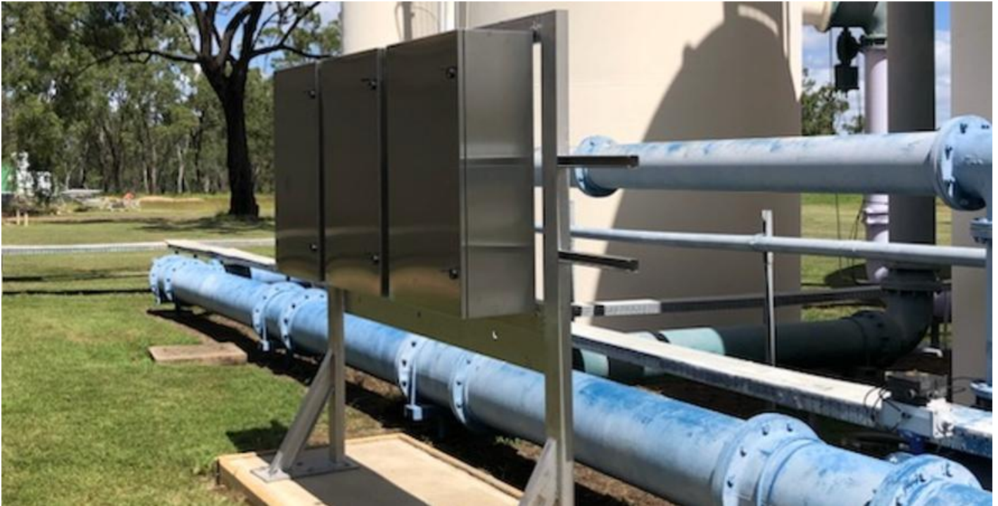
Image 4: Glenden WTP – Installation of Turbidity Analysers underway
